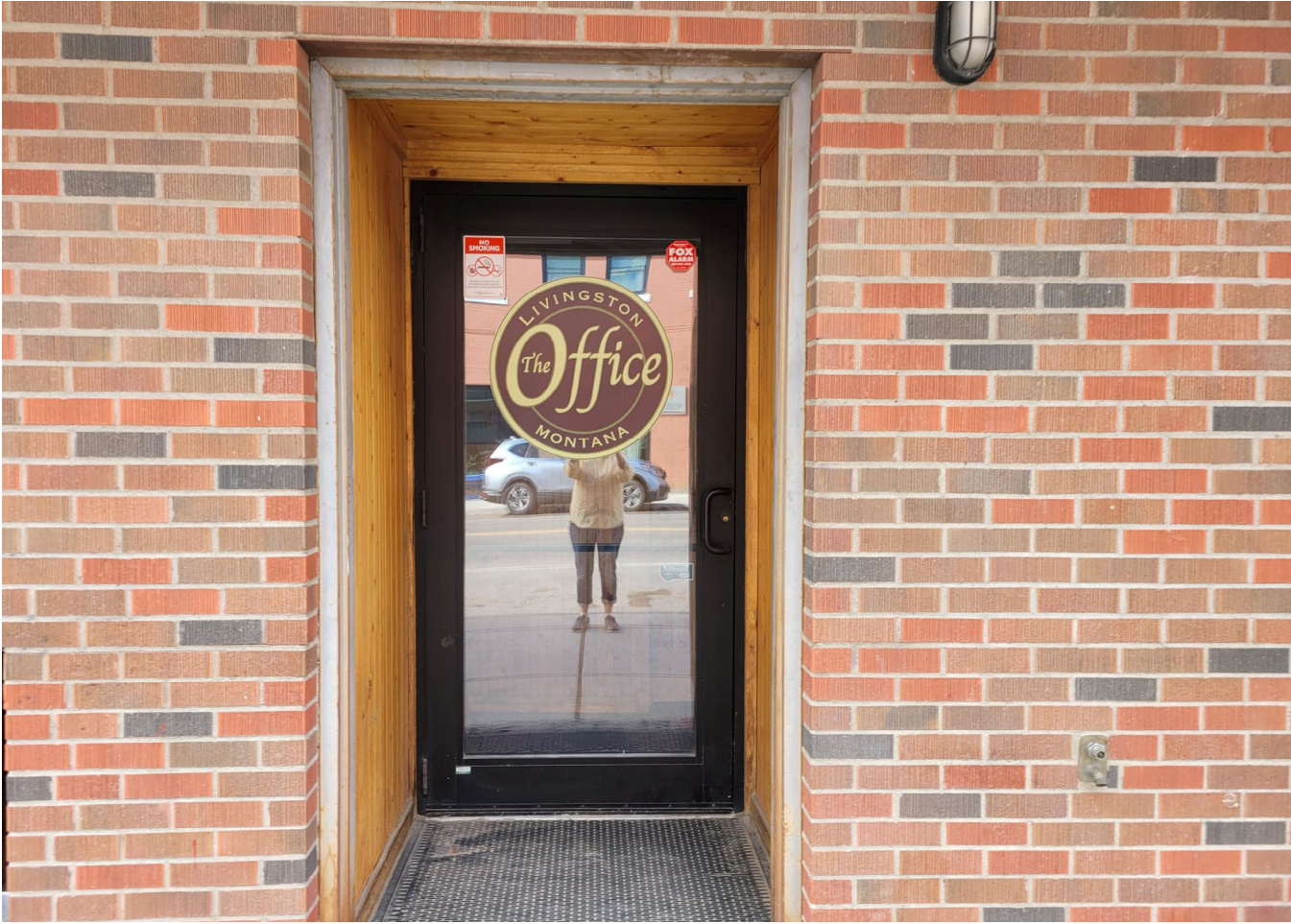
New Side Door Decal (Lewis St) installed Spring 2024
