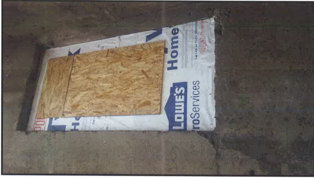
Window Area at Present
