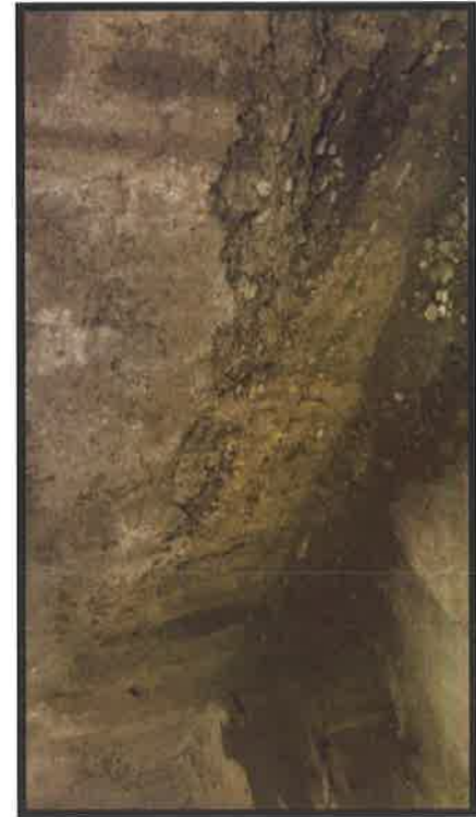
Existing basement wall (facing north) where water drains through the concrete/rock structure during rain and snow events.
