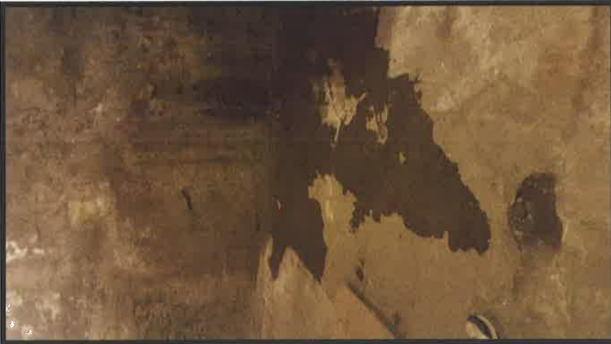
Existing basement wall (facing north) where water drains through the concrete/rock structure during rain and snow events.
