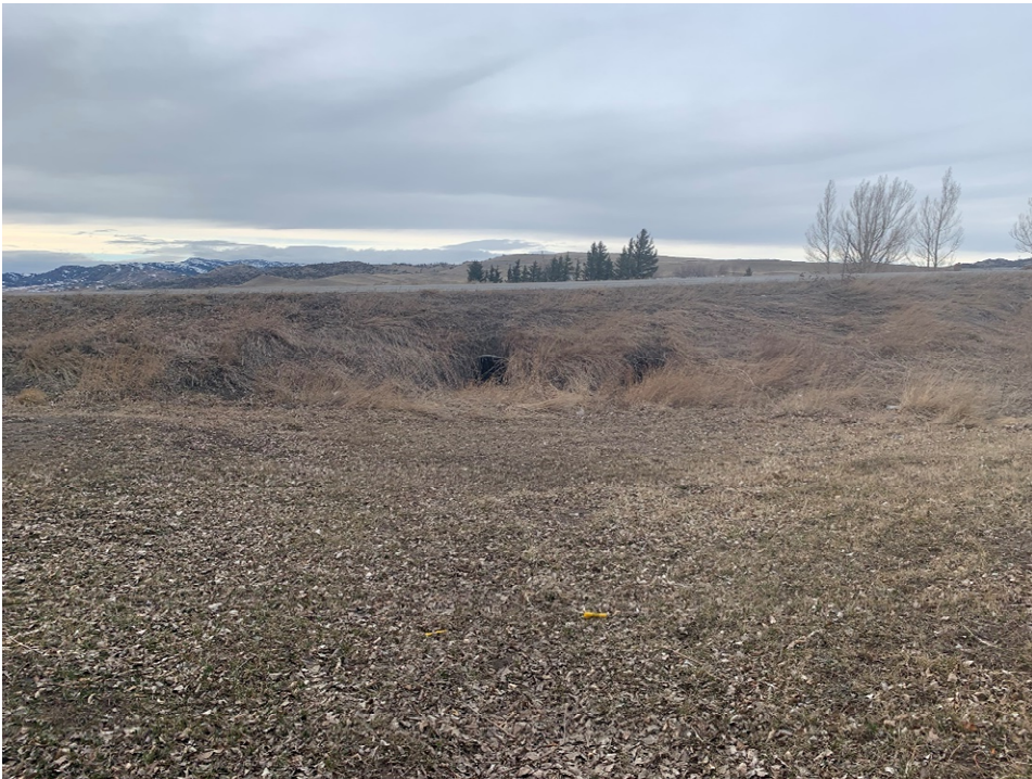
Figure 1: Dual 36” Culverts Looking West (exit of culverts)
