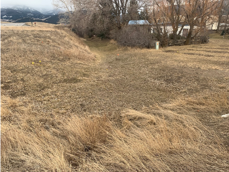
Figure 2: Entrance to Ditch Looking East (exit of culverts behind photographer)
