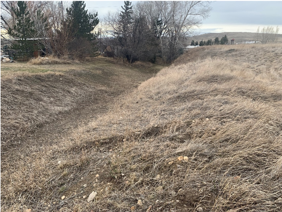
Figure 3: Center of the Ditch Looking West
