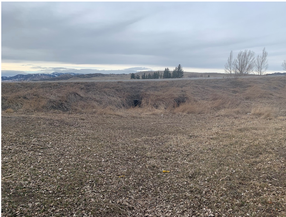
Figure 1: Dual 36” Culverts Looking West (exit of culverts)
