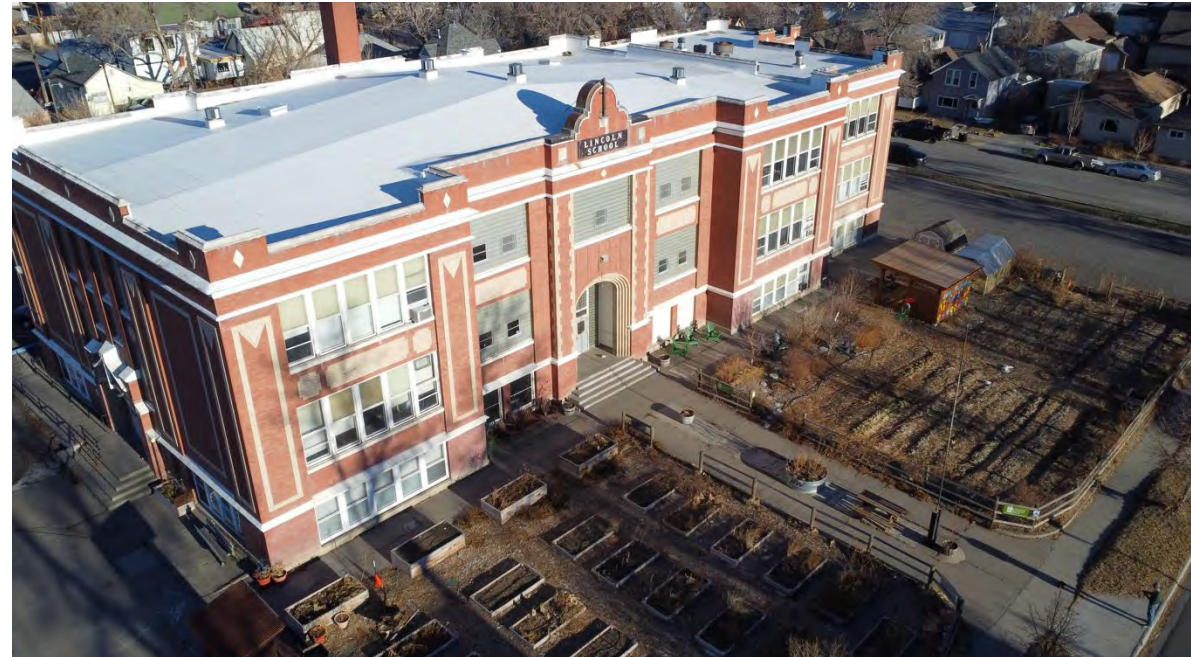
Aerial View of Lewis Street Front of Building with Community Garden and Farm To School Farm
