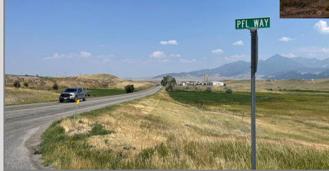
Highway 10 Right of Way
