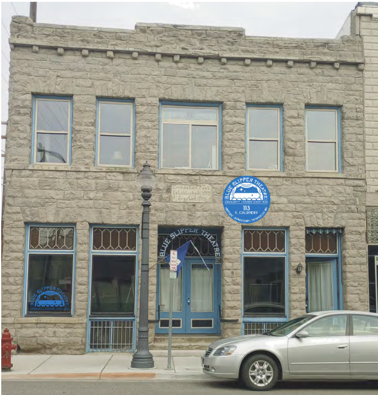
BUILDING: 32 LINEAR FT.
