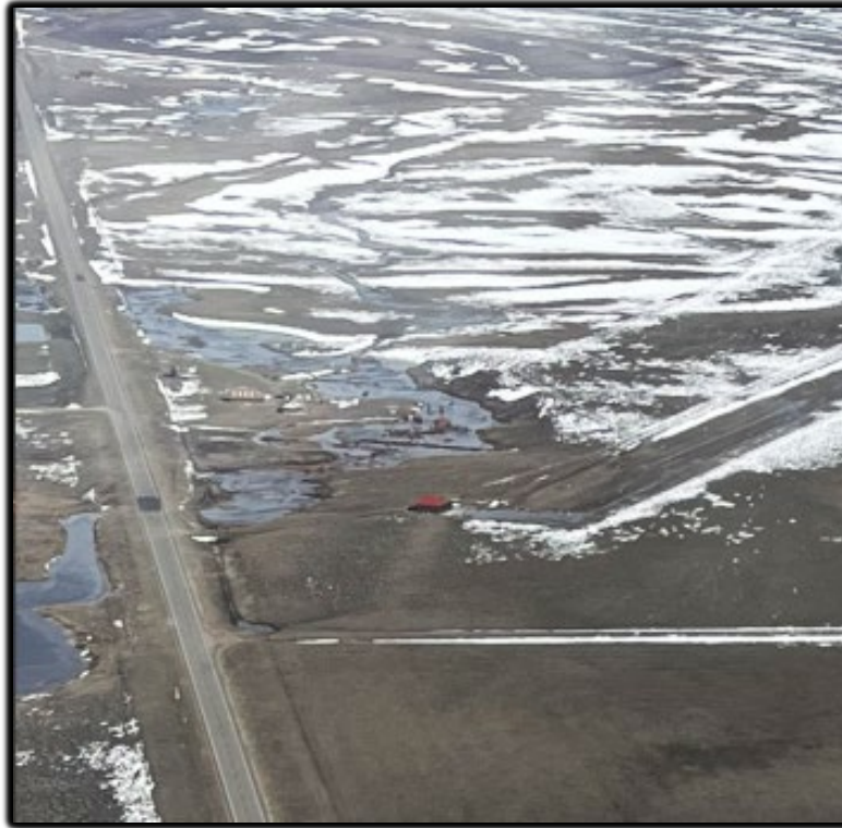
Photograph 3-34 Cottonwood Creek B Flooding 2023 – West of Wilsall Airport along US Highway 89
