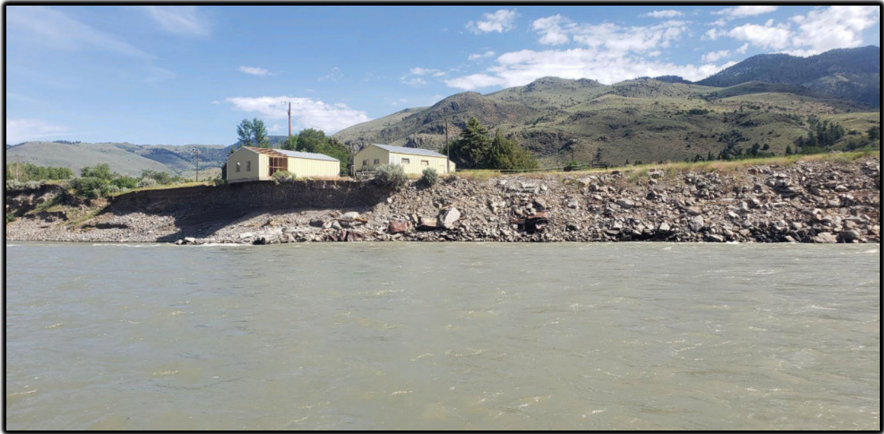
Caption: The Yellowstone River undercut a structure along Highway 89 S near Gardiner, MT during the June 2022 flooding. The structure was still hanging over the edge when the photograph was taken one month after flood waters receded. Source: Pioneer.
