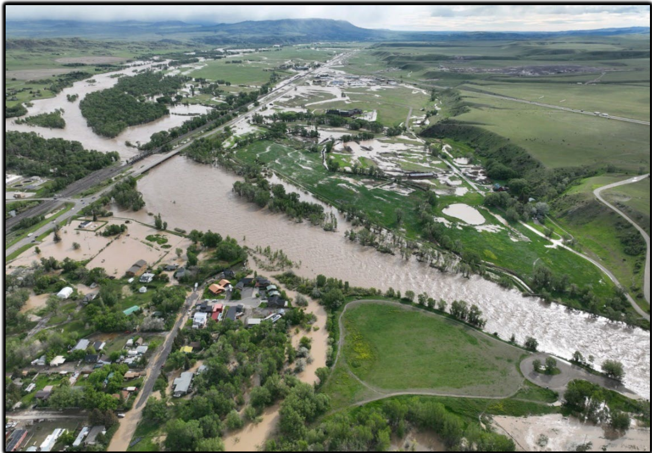
Photograph 3-12 Yellowstone River Flooding 2022 – Livingston, MT Aerial Image
