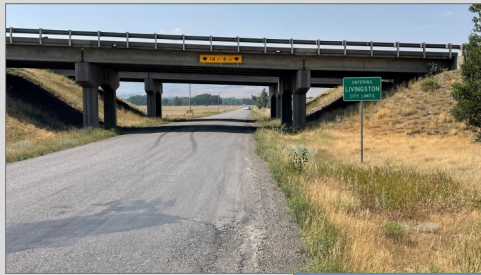
Meyers Lane Underpass
