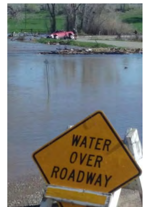
Photo 8. Flooding over roadway at Fiddle Creek Road, Park County, MT.
