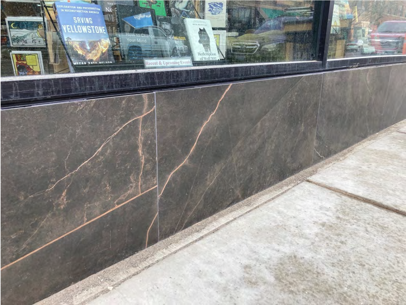
Example of lower tilework bulkhead at 120 S. 2nd St.
