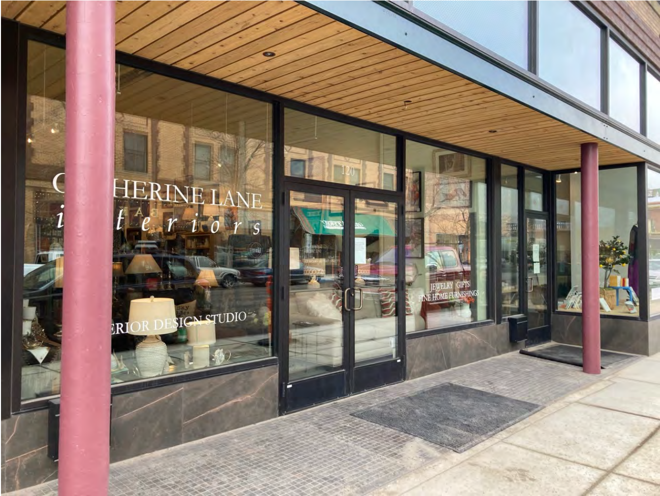
Example of window treatment and of lower tilework bulkhead at 120 S. 2nd St.
