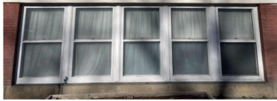
Storm windows installed
