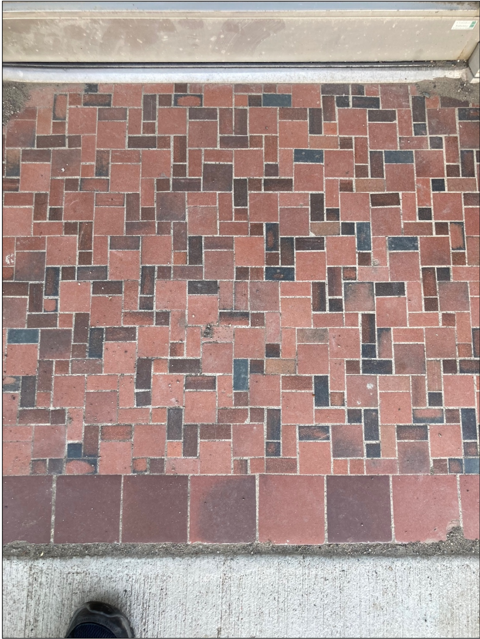
Existing tile entryway of our building This tile will be cleaned and restored if possible. If restoration is not possible, it will be replaced with matching or similar tilework.
