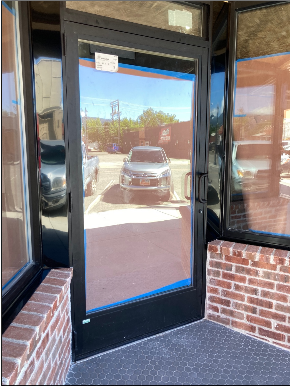
Example of Tubelite mullions and entry door in the 200 block of S. Main Street
