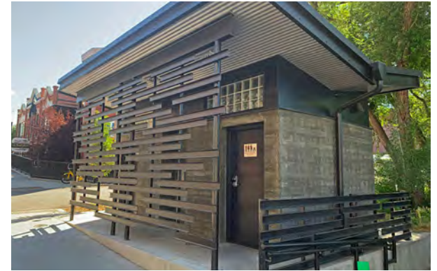
Public Restroom example in Steamboat Springs, CO.
