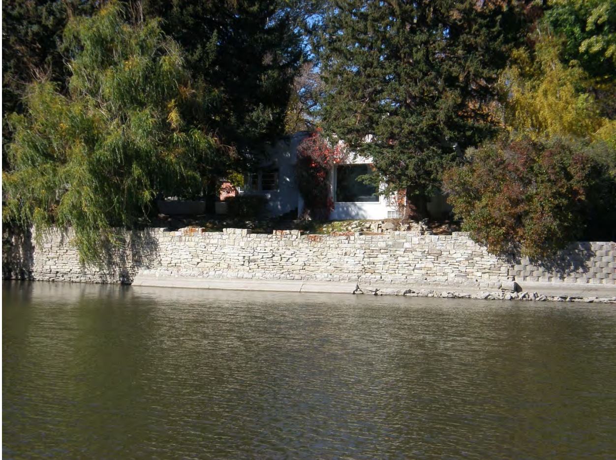
MT_ParkCounty_Sacajawea/Miles Park Historic District_0061 Stone Wall (Resource #36) east of Yellowstone Street Bridge with Lagoon (Resource #26) in foreground. View to the north across the Lagoon.
