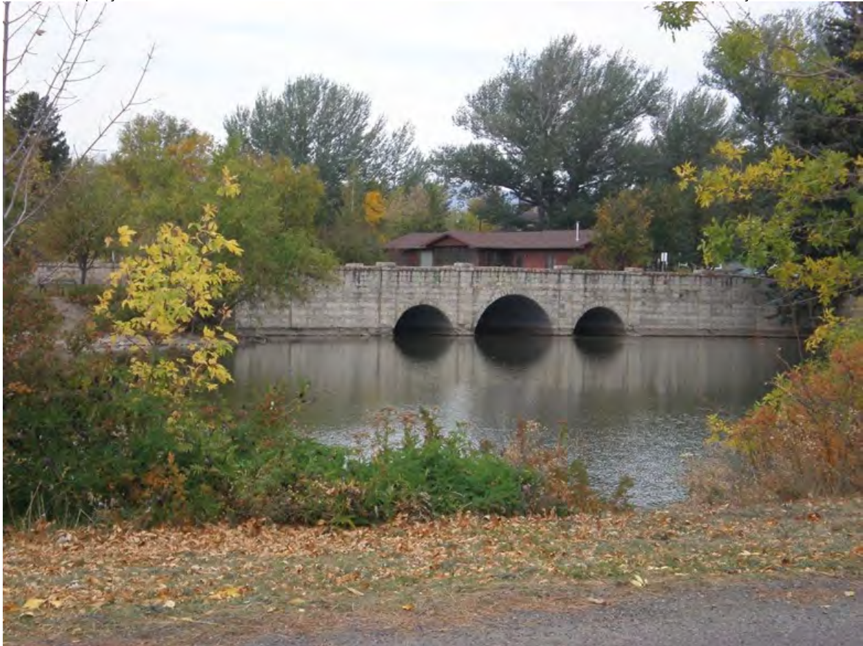
MT_ParkCounty_Sacajawea/Miles Park Historic District_0025 Yellowstone River Bridge (Resource #2). View to the west across the Lagoon (Resource #26) taken from River Drive.
