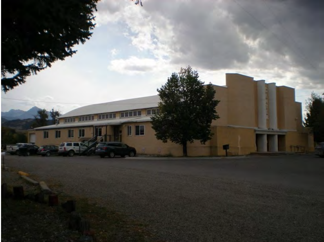
MT_ParkCounty_Sacajawea/Miles Park Historic District_0041 Armory/Civic Center (Resource #21) [east wall and north facade] in Miles Park portion of Sacajawea/Miles Park Historic District. View to the south from River Drive.
