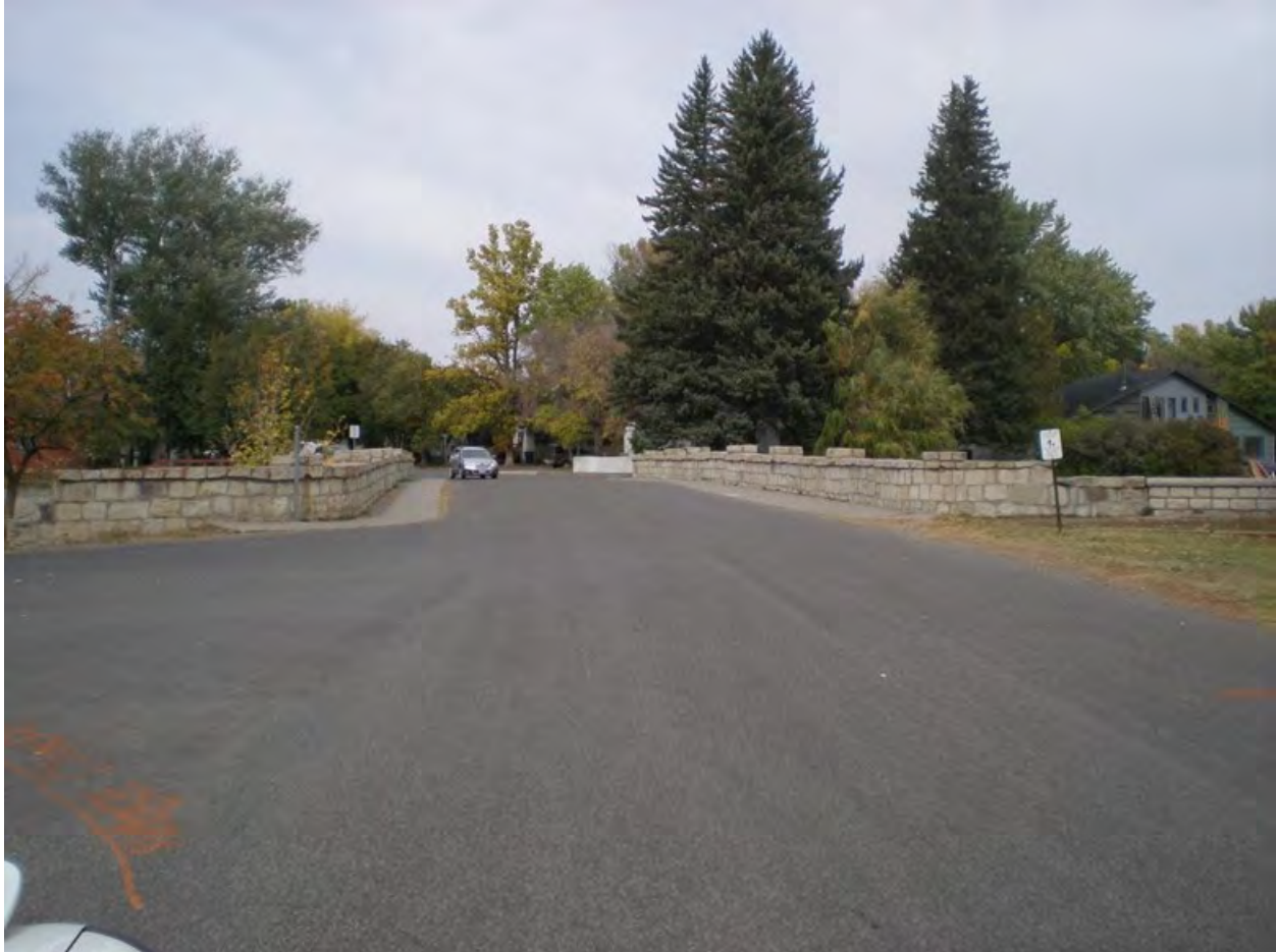
MT_ParkCounty_Sacajawea/Miles Park Historic District_0023 Yellowstone Street Bridge (Resource #2) over the Lagoon to Sacajawea Island portion of the Sacajawea/Miles Park Historic District. View to the north from the intersection of South Yellowstone Street and McGee Drive.
