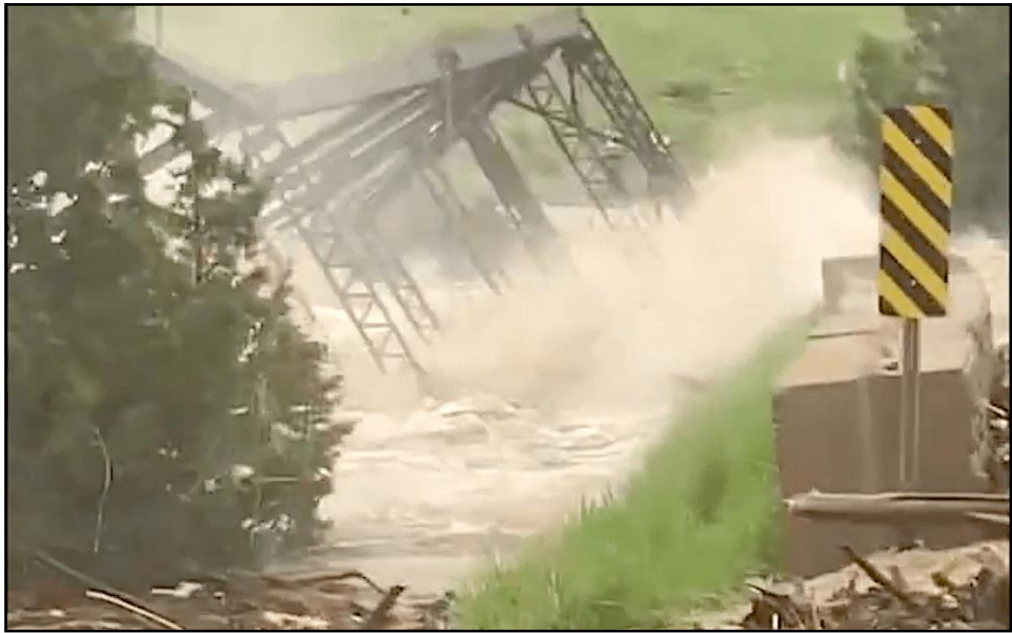
Figure 49. The Carbella Bridge seen as it collapsed into the river (source unknown).
