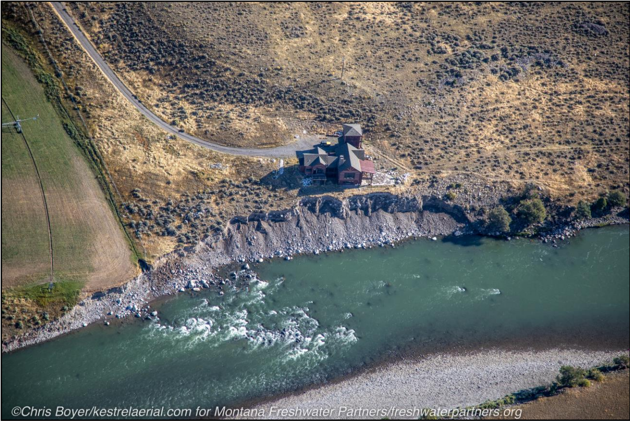
Figure 44. A bankline with a vertical scarp associated with 2022 bankline erosion.
