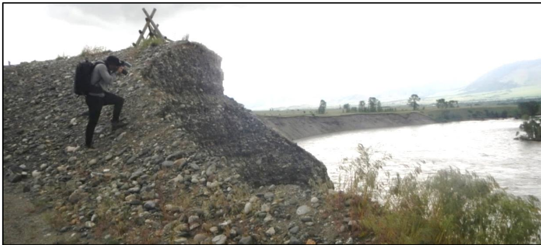
Figure 26. High terrace erosion at Mallards Rest that threatened the access road behind the photographer and resulted in closure.
