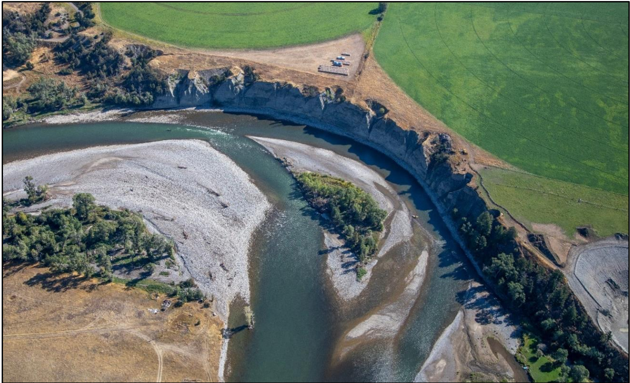
Figure 18. High eroding outwash terrace against river at the Weeping Wall below Pine Creek (Kestral Aerial Services),
