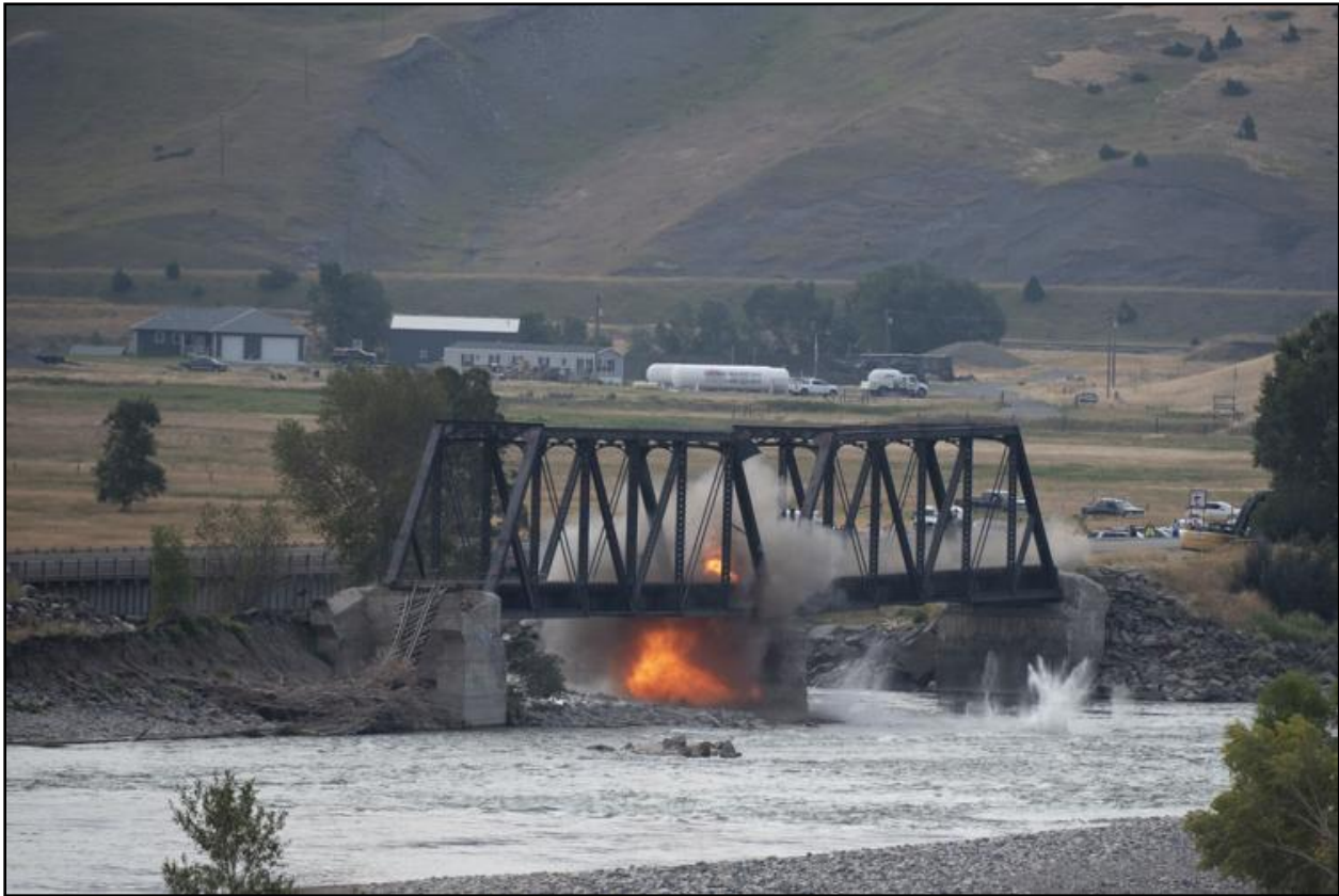
Figure 61. Implosion of the Northern Pacific Railway Bridge on August 24, 2022 (Bozeman Chronicle).
