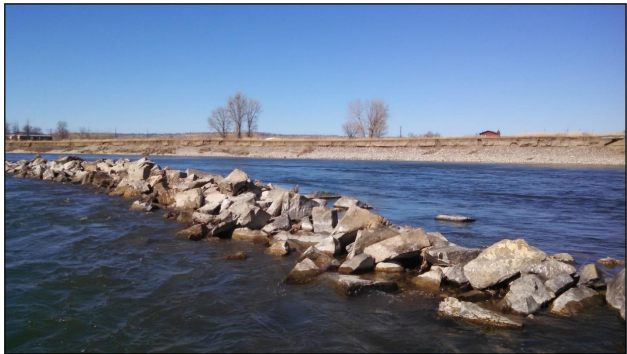
Figure 65. Failed bank armor (2011) in the middle of the Yellowstone River near Park City, MT where the bankline has rapidly eroded back towards the home in the background.
