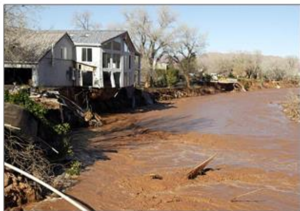
Figure 8. Photos from a 2005 flood event in Saint George Utah, where homes several feet above the mapped floodplain were destroyed by channel migration (originally sourced from Utahfloodrelief.com).
