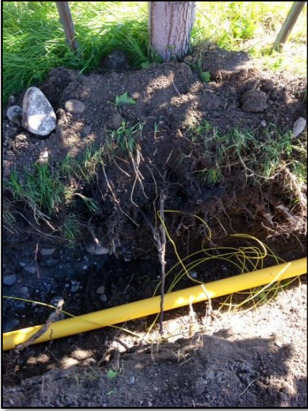
← Dying trees where newer walks were installed. New tree with root damage from 2014 line installation →
