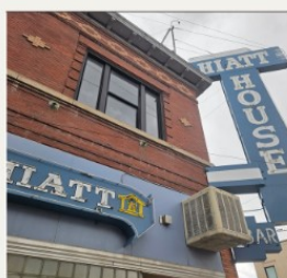
HIATT HOUSE * NEON SIGN REPAINTED
