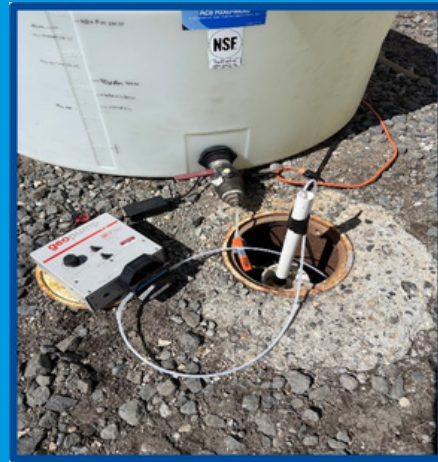
April 2025 - Injecting Sodium Lactate in Well 18-4
