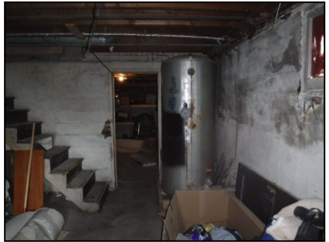
22 : Interior of basement at A1-2
