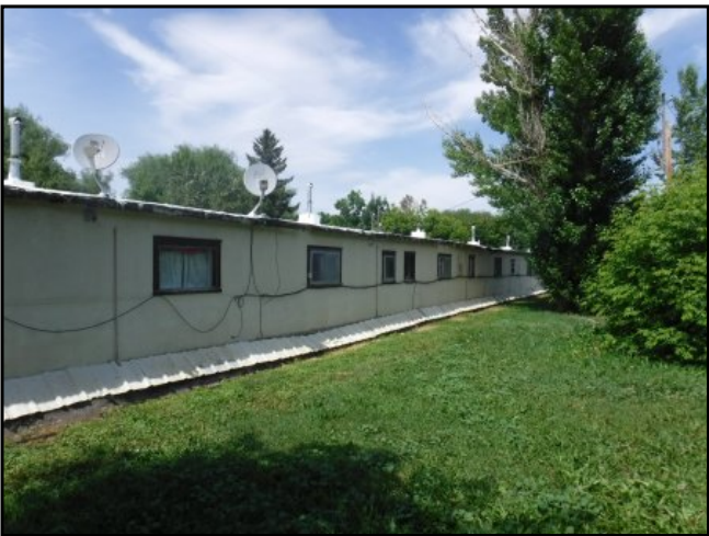
17 : Rear view of the C buildings
