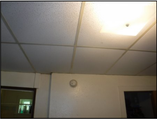
121 : Suspended ceiling system
