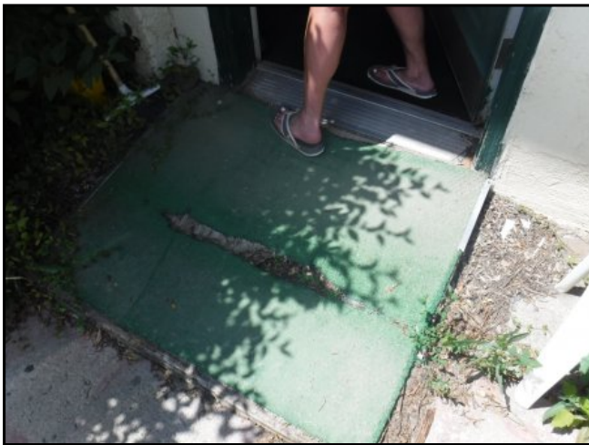
42 : Temporary ramp at unit entry
