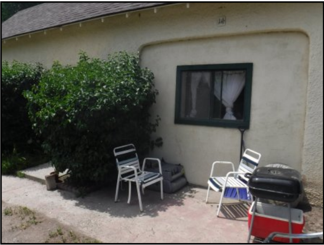
13 : The C buildings were previously provided with carports that have been enclosed.
