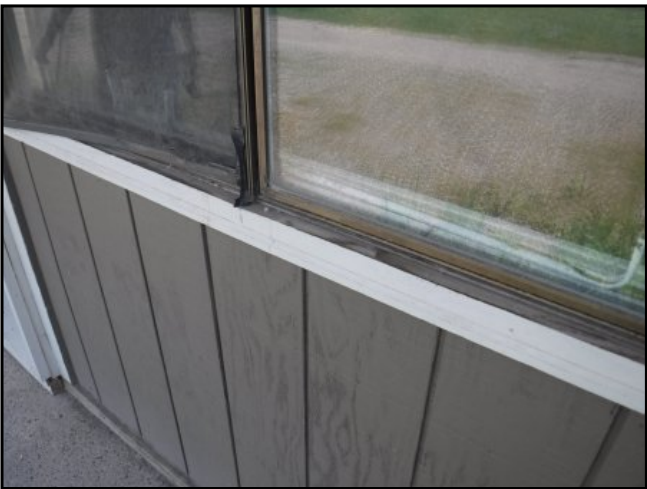
35 : Aluminum framed window assembly
