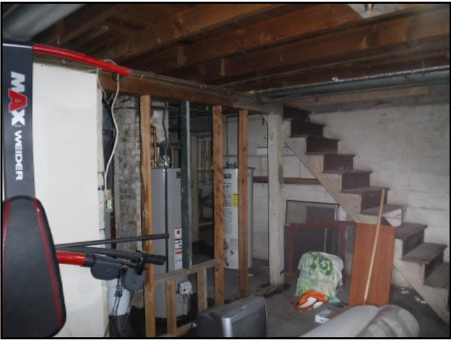
25 : Wood and concrete framing in basement
