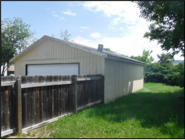
11 : Maintenance building and wood fencing; note the metal roofing at this structure
