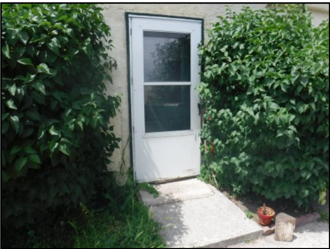
41 : Typical storm door
