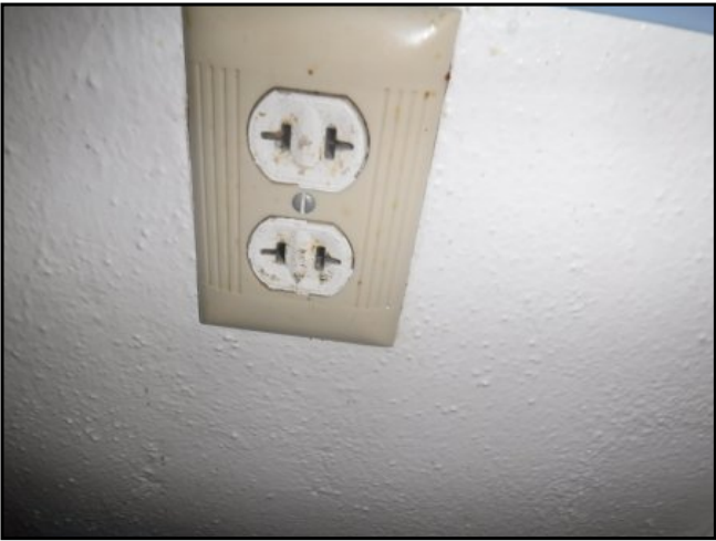
79 : Older outlet noted at the A1-2 builsinf
