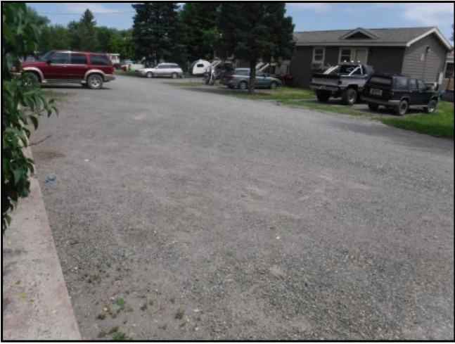
4 : Unpaved road between the C and B buildings.
