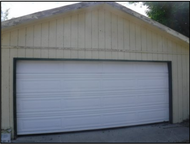
37 : Overhead garage door at the maintenance storage area
