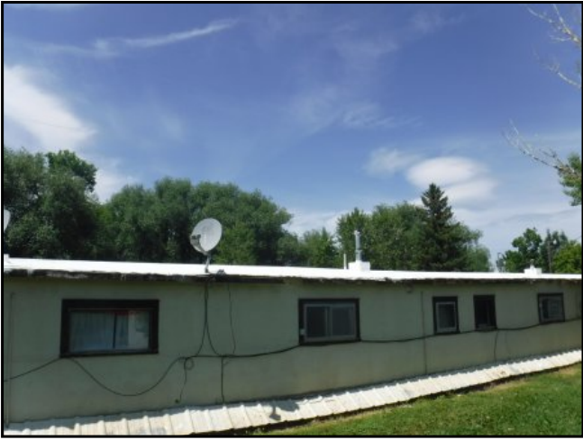
52 : Coated roofing at the rear of A buildings
