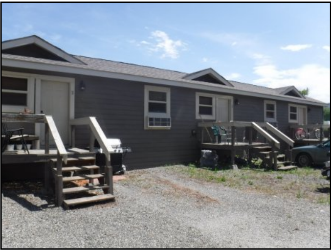
21 : Exterior of the B Building
