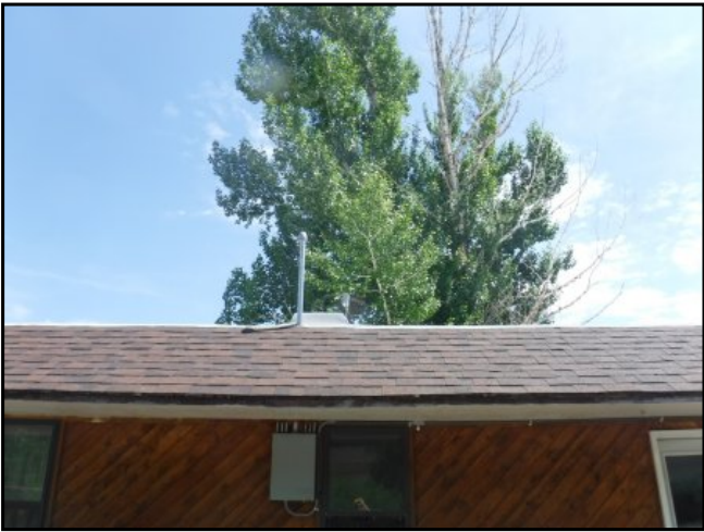
50 : Typical newer asphalt composition shingle roofing
