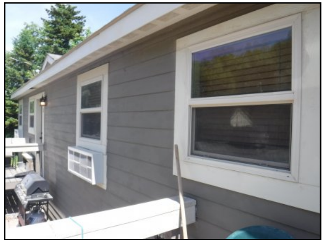
36 : New vinyl windows at the B Building.
