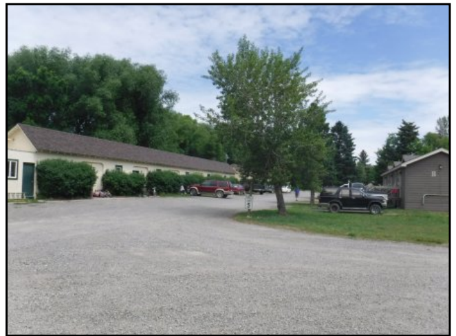
18 : View toward front elevation of A4-12
