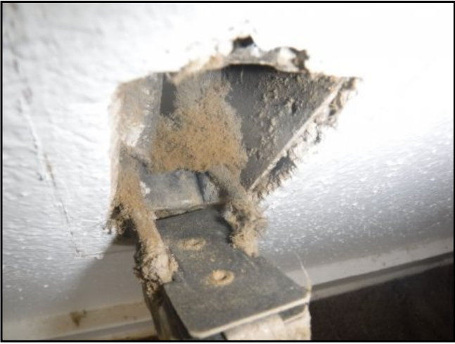
81 : Original wiring at the A 1-2 building
