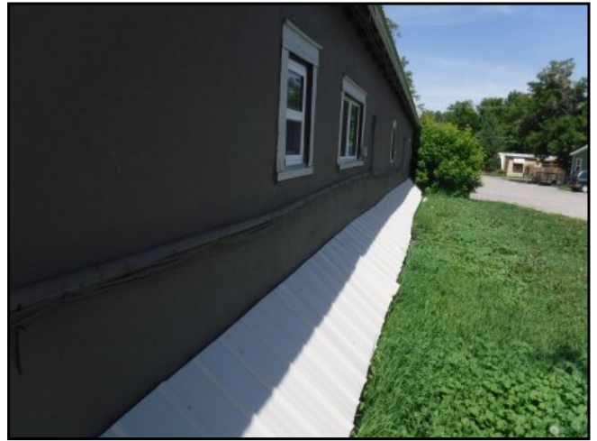
20 : Rear view of the C buildings
