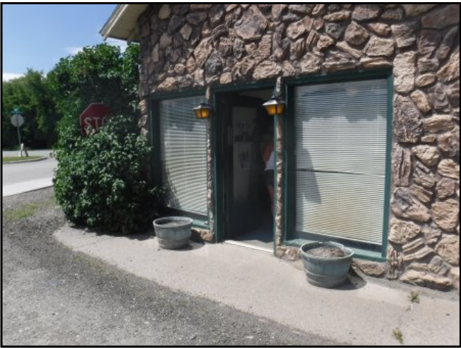
39 : Entry to the leasing office. Note the stone veneer, wood windows and wood entry door
