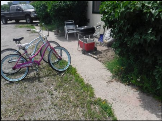
6 : Typical pedestrian walkway.
