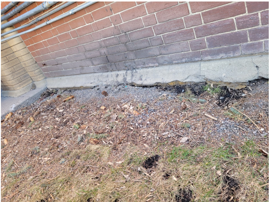
Figure 6: Improper drainage at the Livingston Depot Beanery Building. According to the National Park Service Preservation Brief, “Holding the Line: Controlling Unwanted Moisture in Historic Buildings,” effective exterior drainage and eliminating low spots around building foundations is paramount to protecting historic structures.
