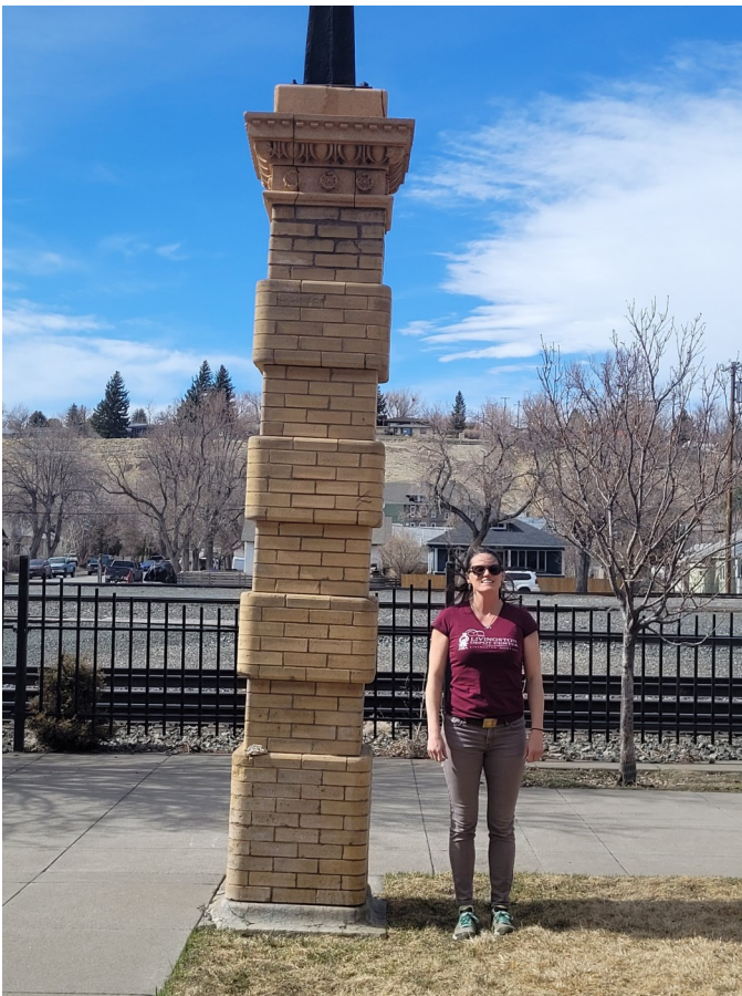
Figure 2: Tilting light stanchion due to settling. The Depot will conduct minor structural stabilization to re-level a light stanchion in the courtyard that is independent of any other structure.
