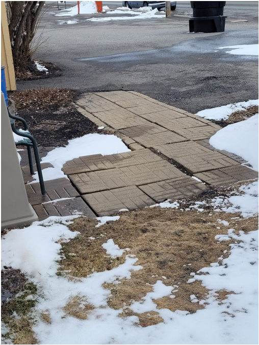
Figure 7: Improper drainage at the Livingston Depot Beanery Building. Appropriately graded concrete will reduce water seepage into the foundation of historic structure, improve accessibility for persons with disabilities, and reduce blight.
