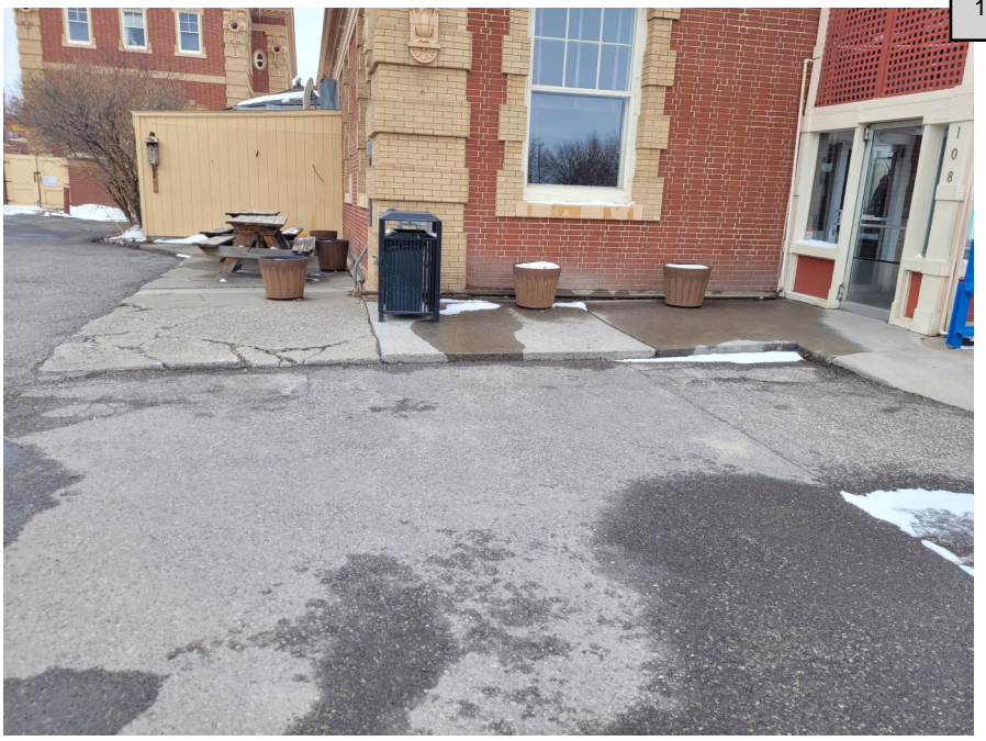
Figure 7: Improper drainage at the Livingston Depot Beanery Building. Appropriately graded concrete will reduce water seepage into the foundation of historic structure, improve accessibility for persons with disabilities, and reduce blight.
