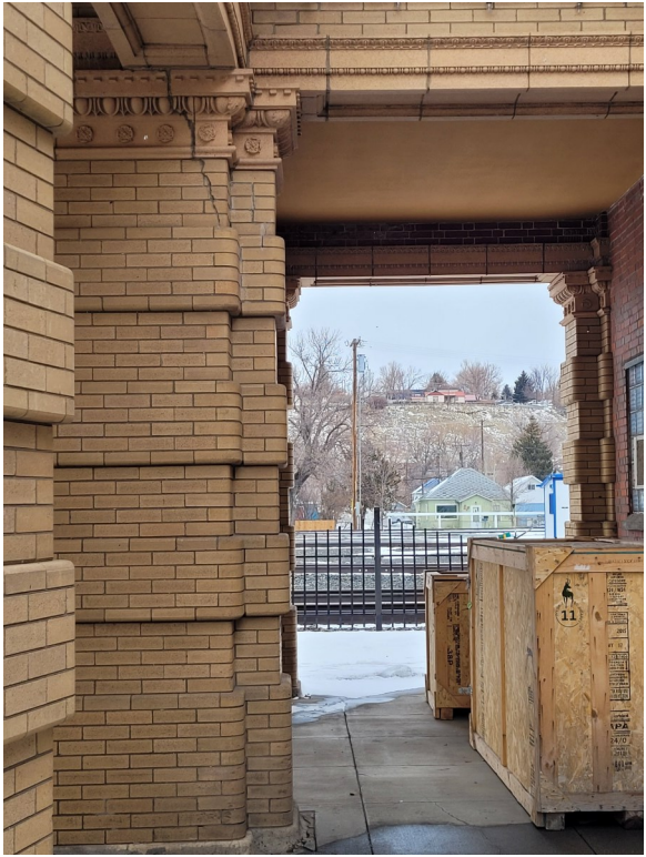
Figure 5: Improper drainage at the Livingston Depot Beanery Building. Pooling runoff is causing significant deterioration of the brick and some settling of the columns. (The Depot Foundation fixed cracks in the colonnade during the 2016 Save America’s Treasures “Roof Project;” but did not address the drainage issues.) Filling this area with an appropriately graded concrete slab will reduce deterioration of the original brick façade and maintain the structural integrity of the colonnade.
