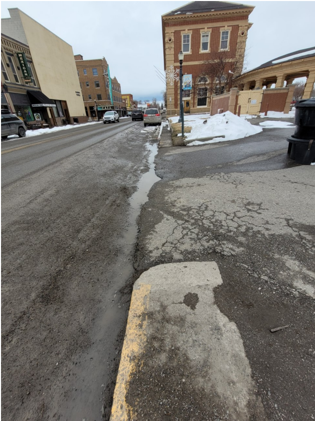
Figure 8: Potholes causing damage to sewer lines. The owners of the Northern Pacific Beanery generously provide after-hours parking for their neighbors and their customers. Unfortunately, this increased use has caused large potholes at the entrance and exit to the parking lot. Not only are the potholes unsightly, vehicles are causing slumping in the sewage pipes below. Installation of appropriate concrete aprons will prevent future
