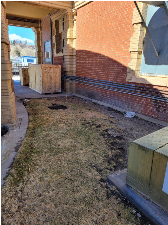
Figure 5: Improper drainage at the Livingston Depot Beanery Building. Pooling runoff is causing significant deterioration of the brick and some settling of the columns. (The Depot Foundation fixed cracks in the colonnade during the 2016 Save America’s Treasures “Roof Project;” but did not address the drainage issues.) Filling this area with an appropriately graded concrete slab will reduce deterioration of the original brick façade and maintain the structural integrity of the colonnade.
