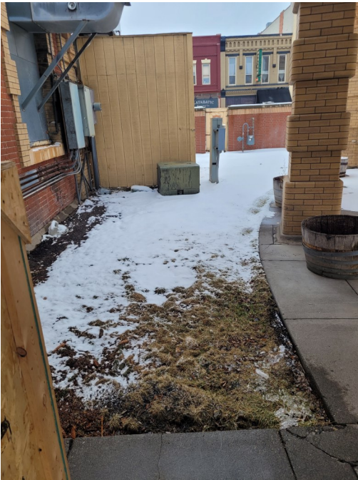
Figure 6: Improper drainage at the Livingston Depot Beanery Building. According to the National Park Service Preservation Brief, “Holding the Line: Controlling Unwanted Moisture in Historic Buildings,” effective exterior drainage and eliminating low spots around building foundations is paramount to protecting historic structures.
