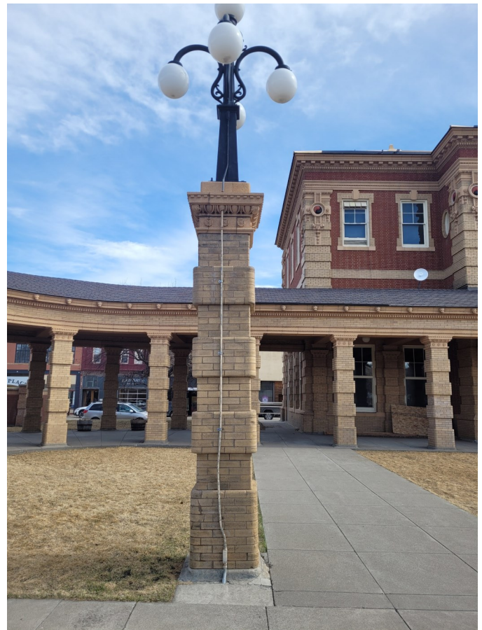
Figure 2: Tilting light stanchion due to settling. The Depot will conduct minor structural stabilization to re-level a light stanchion in the courtyard that is independent of any other structure.
