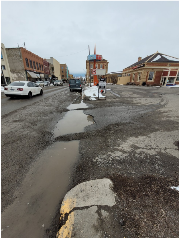
Figure 8: Potholes causing damage to sewer lines. The owners of the Northern Pacific Beanery generously provide after-hours parking for their neighbors and their customers. Unfortunately, this increased use has caused large potholes at the entrance and exit to the parking lot. Not only are the potholes unsightly, vehicles are causing slumping in the sewage pipes below. Installation of appropriate concrete aprons will prevent future
