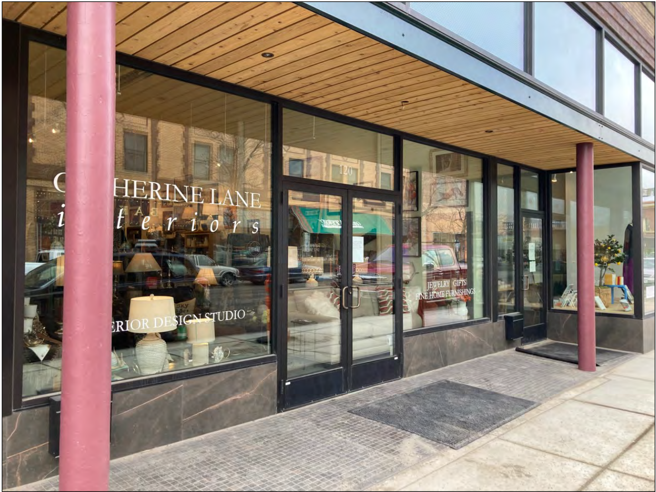
Example of the window treatment, the mullions and the lower tilework bulkhead at 120 S. 2nd St. Our renovation at 116 S. Main will be quite similar in style.
