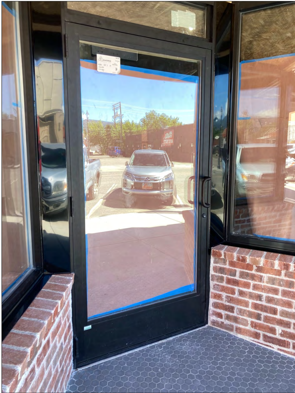
Example of Tubelite mullions and entry door in the 200 block of S. Main Street
