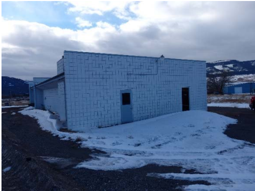
North elevation facing Sun Avenue.
