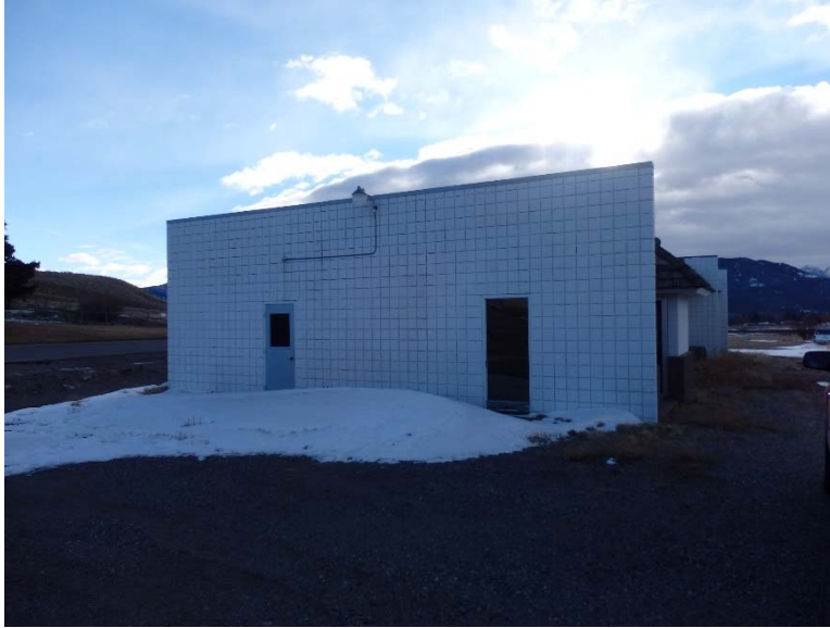
North elevation, 01/12/2016, CCS.
