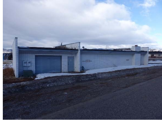
East elevation facing Star Road.
