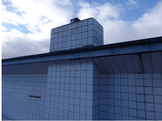
Soffit and chimney close-up.
