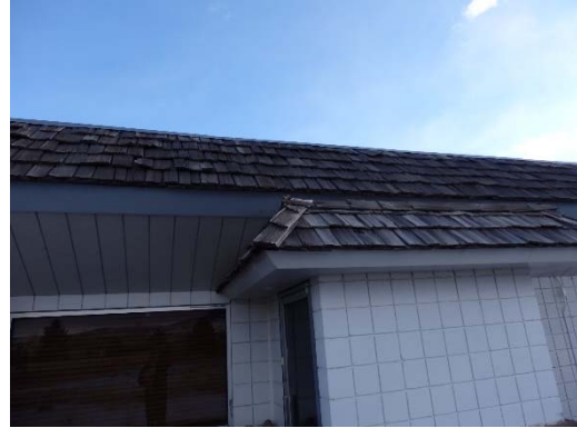
Cedar roof apron close-up.
