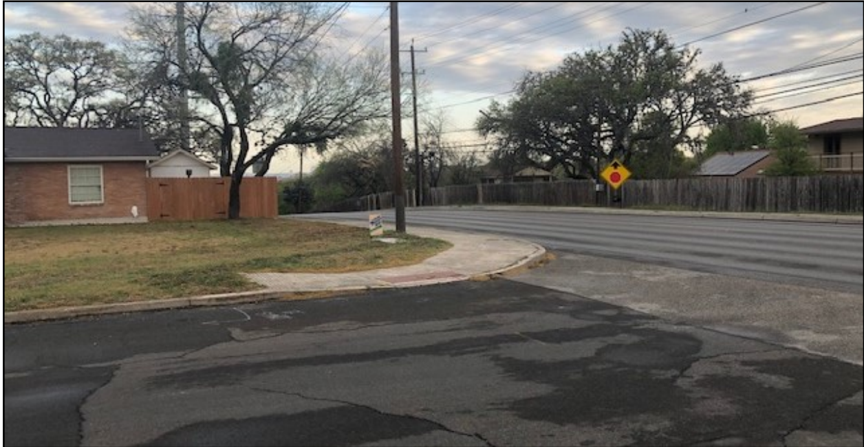
Figure 6. Wooden Fence Obstruction on South-West Corner of Intersection
