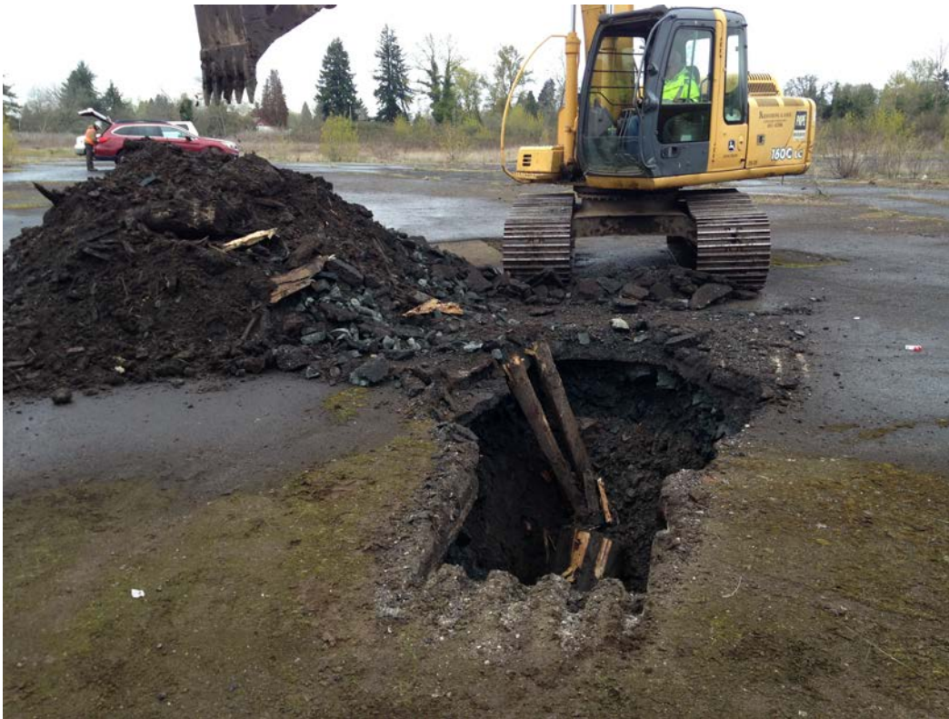
Photo 4A. Wood debris being removed from TP-3
