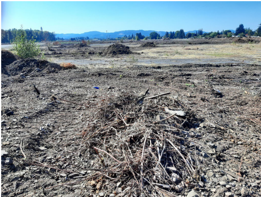
Photo 1. Push piles and heavy equipment tracks viewed from the north end of the project at the approximate east-west midpoint. The view is towards the south. Photo taken September 21, 2023.
