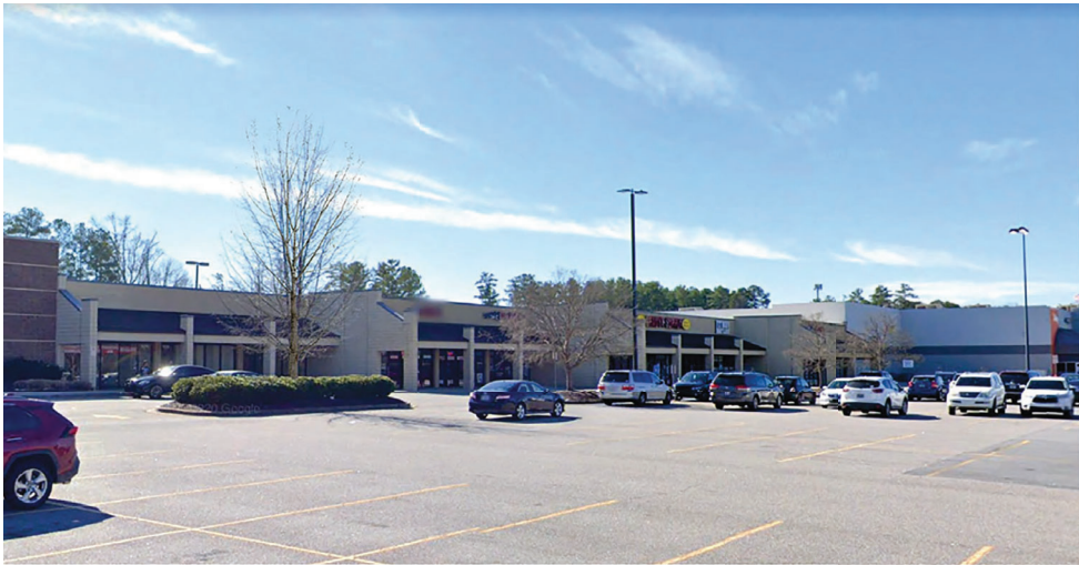
Lawrenceville Crossing Shopping Center Outparcel 2 (Existing Conditions)
