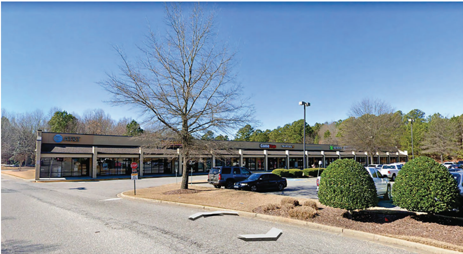
Lawrenceville Crossing Shopping Center Outparcel (Existing Conditions)
