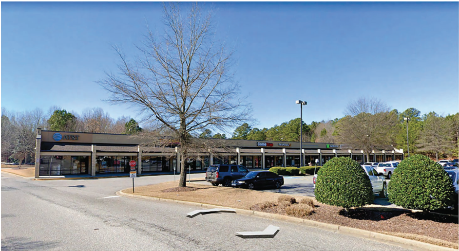
Lawrenceville Crossing Shopping Center Outparcel (Existing Conditions)
