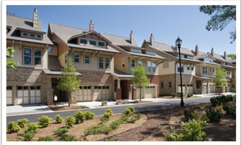
Ex. No. 2 - Front Entry Townhouse Dwelling Units
