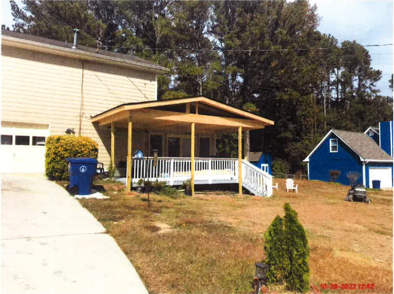
CEU2022-06441_432 NEW HOPE RD_5173 025_RIGHT SIDE OF HOME ADDITION_10262022
