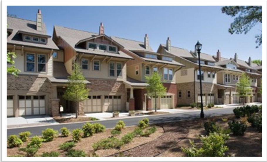
Ex. No. 2 Front Entry Townhouse Dwelling Units
