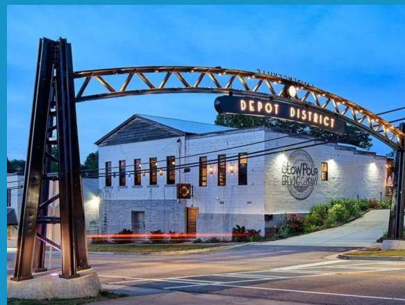
Gateway Signage Lawrenceville, GA
