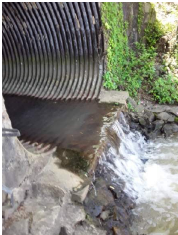
Picture 1: Downstream headwall.
