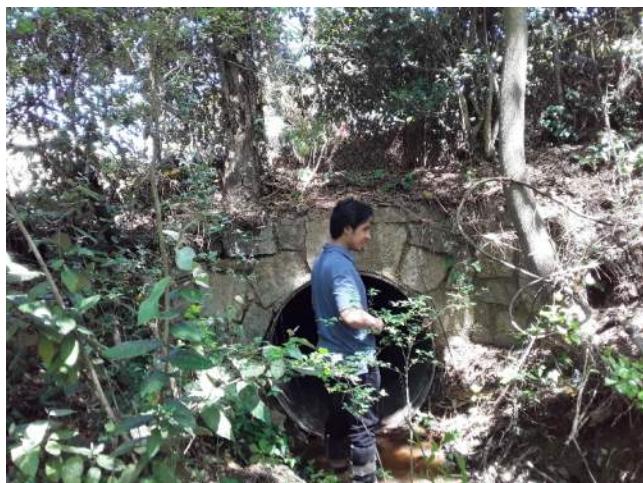
Picture 1: Upstream headwall.
