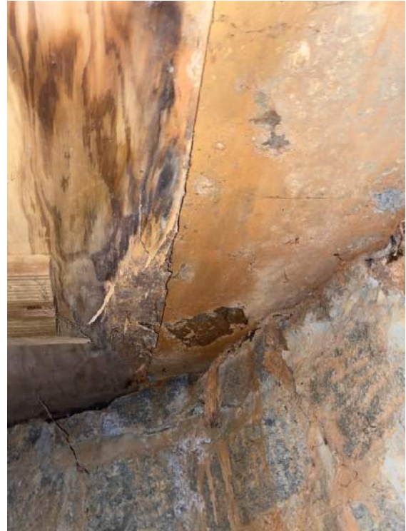
Picture 6: Concrete slab as roof of junction box. Wood forms remain across structure.
