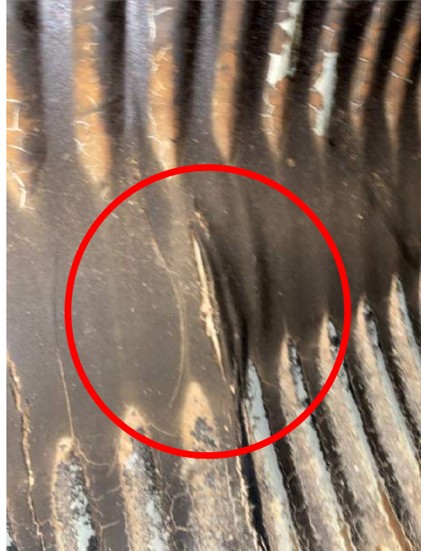
Picture 12: Small crease on pipe that seems to be cracked close to downstream headwall.
