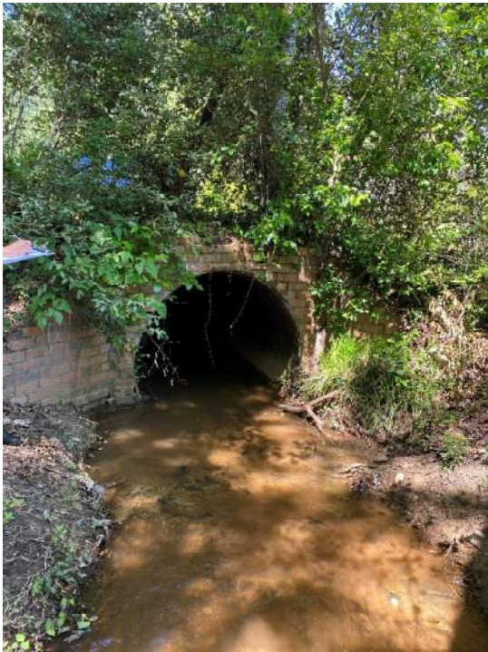
Picture 1: Upstream headwall
