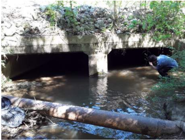
Picture 1: Upstream Headwall
