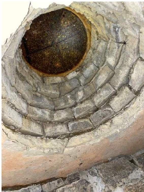
Picture 7: Customized junction box structure where the pipe turns.
