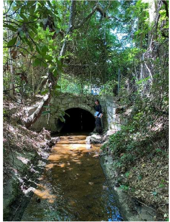
Picture 13: Upstream headwall
