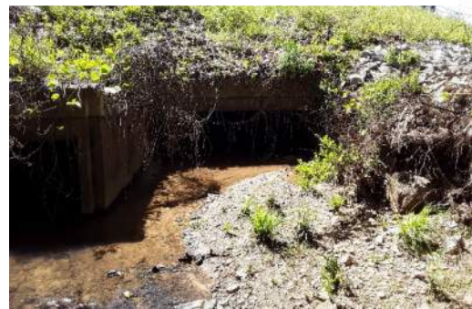
Picture 5: Right downstream headwall
