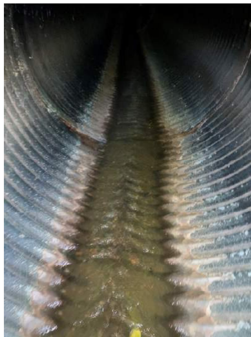
Picture 2: Bottom is slightly corroded but solid.
