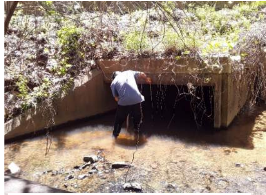
Picture 4: Left downstream headwall
