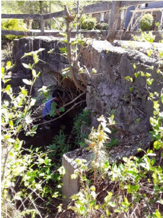
Picture 1: Downstream headwall
