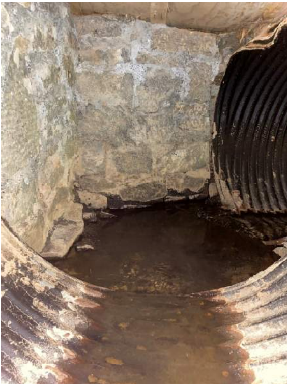
Picture 9: Customized junction box where pipe turns.
