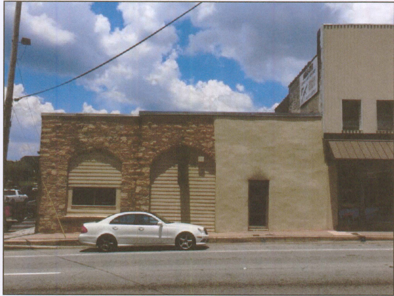
EXISTING SOUTH (FRONT) FACADE
