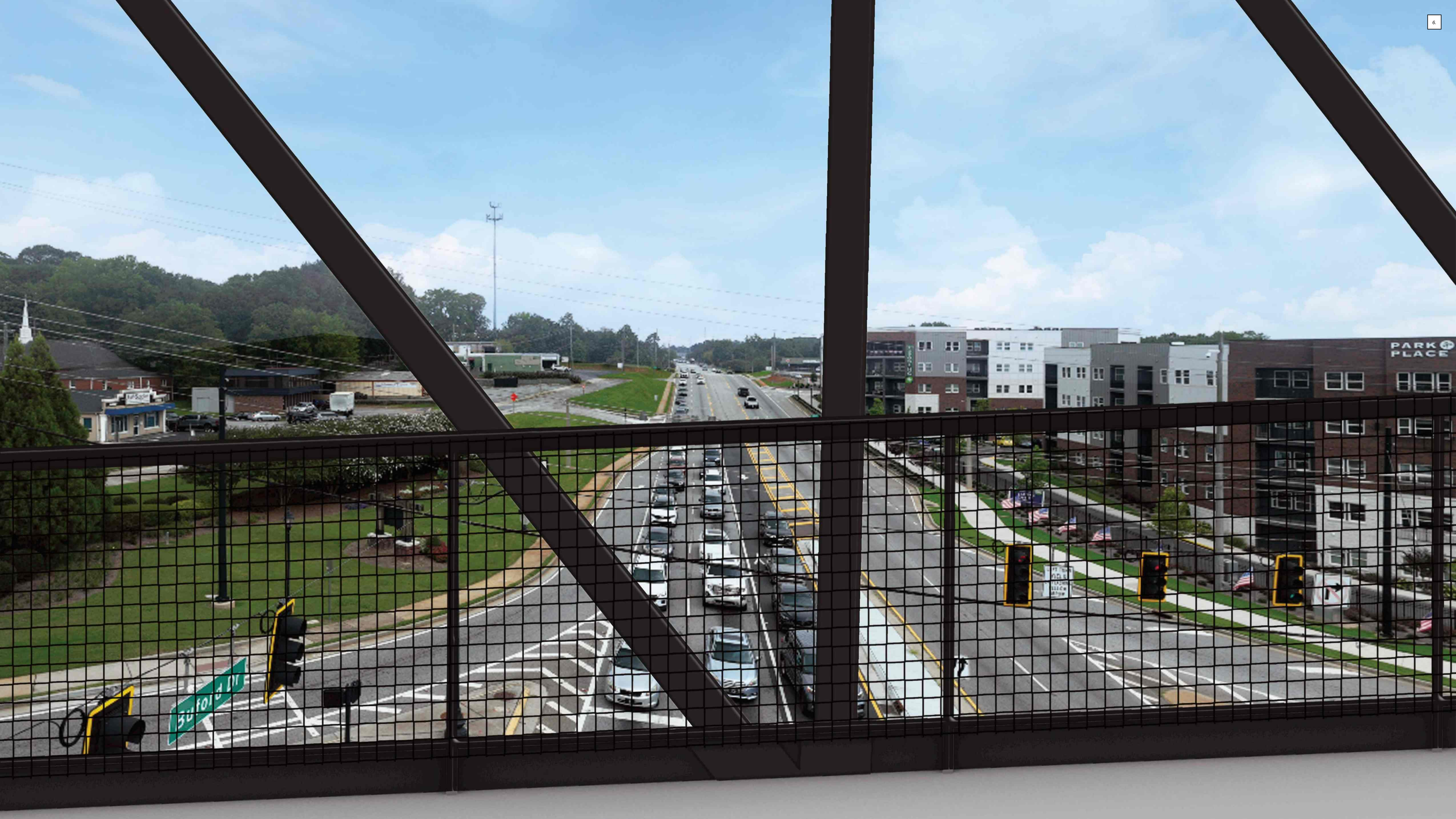
DRONE IMAGERY | BUFORD DRIVE PEDESTRIAN BRIDGE | VIEW NORTH
