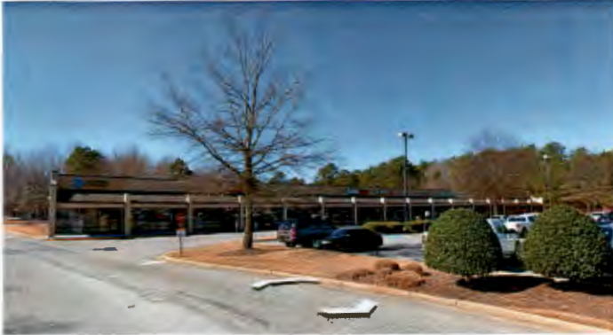
Lawrenceville Crossing Shopping Center Outparcel (Existing Conditions)
