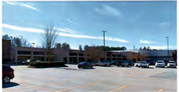
Lawrenceville Crossing Shopping Center Outparcel 2 (Existing Conditions)
