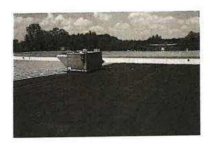
EPDM is an extremely durable synthetic rubber roofing membrane that is used worldwide. EPDM is available in both black and white and is sold in a variety of widths and thicknesses. Its superior durability and cost-effectiveness are part of what makes EPDM one of the most popular flat roof systems installed in the U.S. today.
