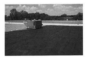
EPDM is an extremely durable synthetic rubber roofing membrane that is used worldwide. EPDM is available in both black and white and is sold in a variety of widths and thicknesses. Its superior durability and cost-effectiveness are part of what makes EPDM one of the most popular flat roof systems installed in the U.S. today.
