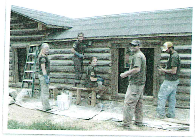
Example of Building Restoration
