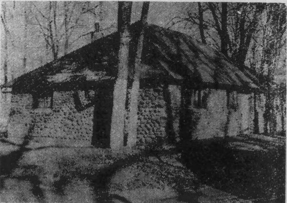
1936 May 27 Laurel Outlook . Two new buildings at Riverside Park by May of 1936. Top: Riverside Hall / Jaycee Building prior to the cobblestone veneer work done in the summer of 1936. Bottom: East end of the future Rifle Club building.
