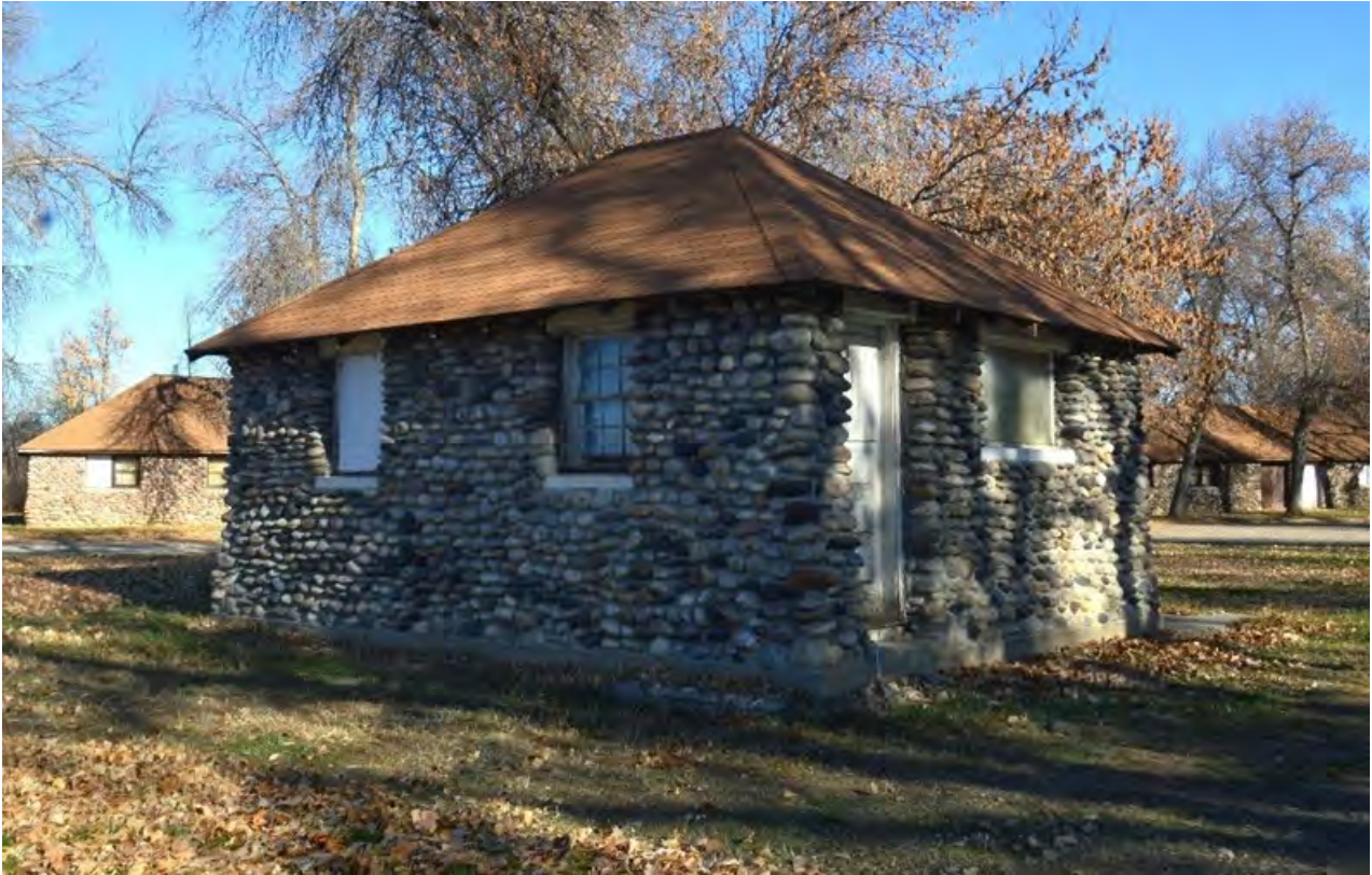
MT_YellowstoneCounty_RiversidePark_0010. Small River Rock Building / Guards' Building, looking north (Rifle Club building is in the background). November 20, 2023.
