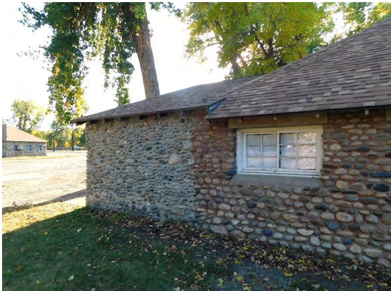
MT_YellowstoneCounty_RiversidePark_0013. American Legion Hall / Bath House, looking southwest at add-on façade from the 1950s (left) marked by color change in mortar. October 07, 2023.
