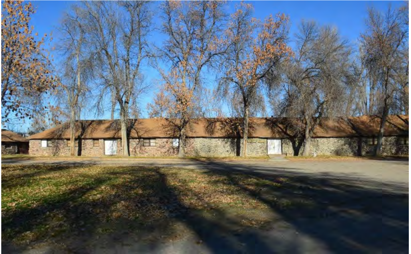
MT_YellowstoneCounty_RiversidePark_0016. Rifle Club building, looking north. November 20, 2023.
