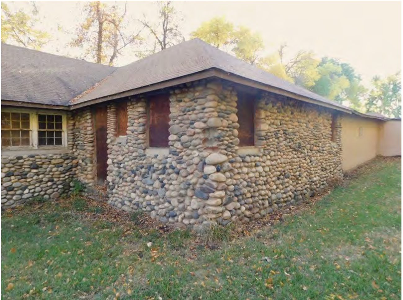
MT_YellowstoneCounty_RiversidePark_0017. Rifle Club building, view looking southwest. October 07, 2023.
