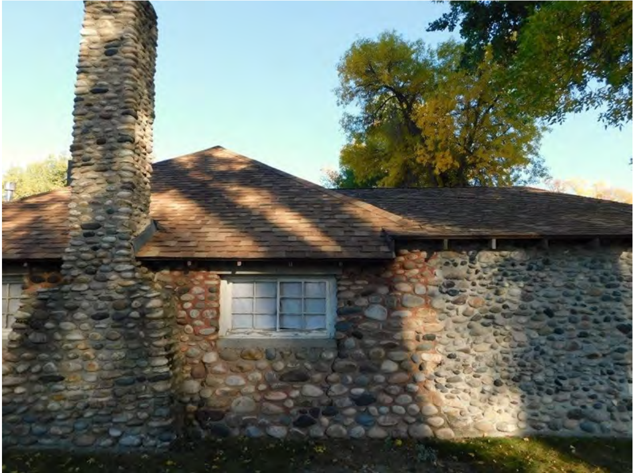
MT_YellowstoneCounty_RiversidePark_0014. American Legion Hall / Bath House, looking east at chimney and front façade (right) marked by color change in mortar. October 07, 2023.
