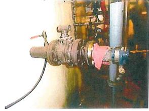
All welded is to be cleaned and re-coated.
