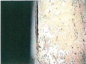
3. Weld patch over hole in the Methane Box.
