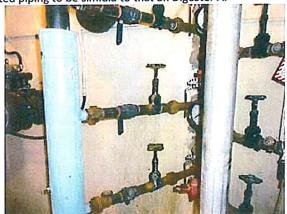
6. Remove valve, grout inside of 4-inch pipe and cap pipe.
