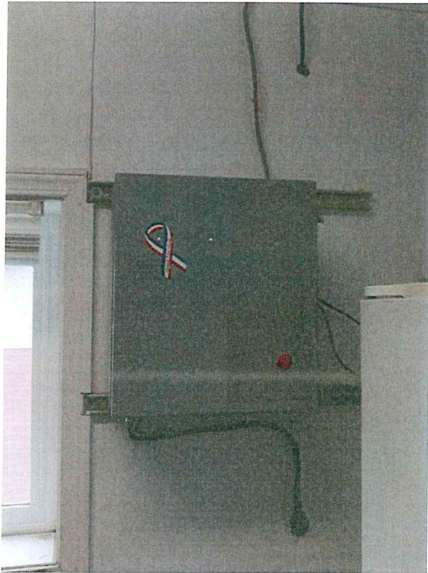
RP and TPP VFD Replacements in the Low Service Building.
