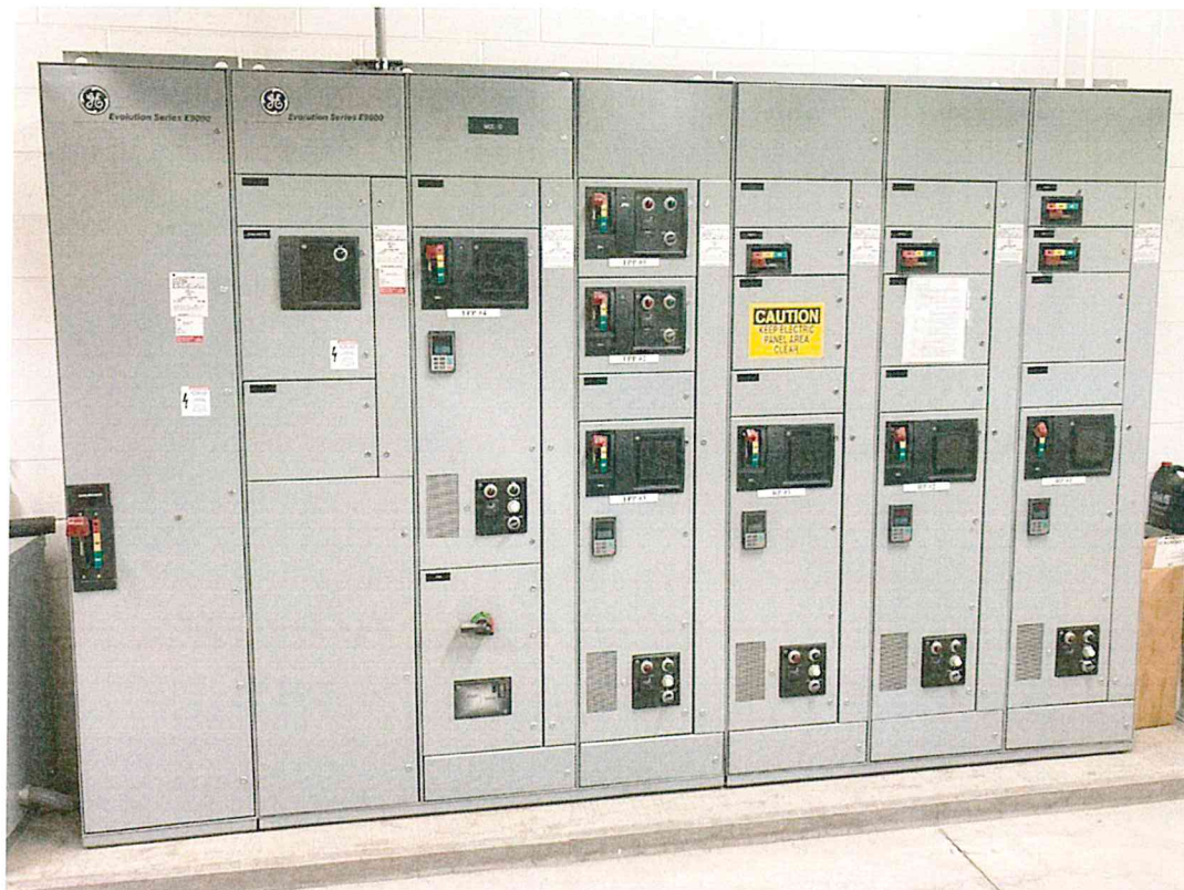
RP and TPP VFD Replacements in the Low Service Building.
