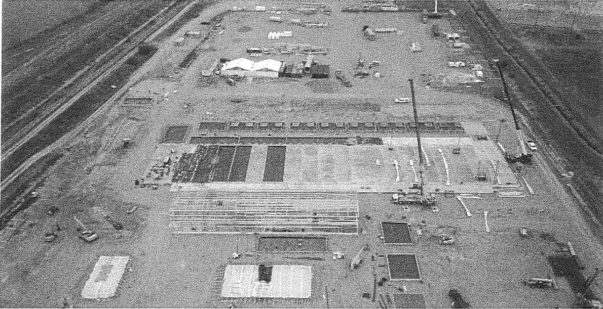
Source: Galvan Decl., Ex. 13 (Photo of NorthWestern Energy Laurel gas plant construction (Nov. 8, 2022))
