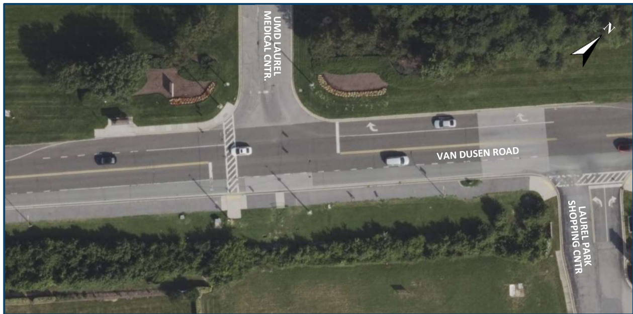
Figure 3 VAN DUSEN ROAD AT UMD LAUREL MEDICAL CENTER
