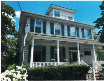
VIEW FROM FRONT/SOUTHWEST CORNER OF THE HOUSE
