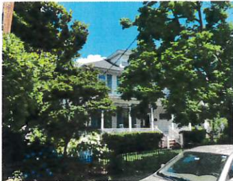
VIEW FROM FRONT/SOUTHWEST CORNER OF THE HOUSE
