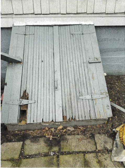
Photo of current cellar door that may be removed:
