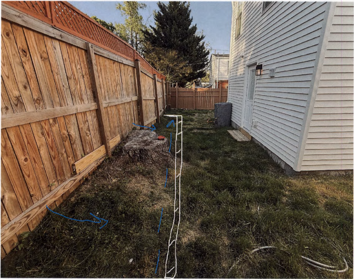
Figure 4: Stormwater that enters downslope through or under the fence will be caught by the garden and stone wall, then diverted downslope to a gravel drain away from the foundation. The existing stump will stay in place and become a garden feature “flower pot”.
