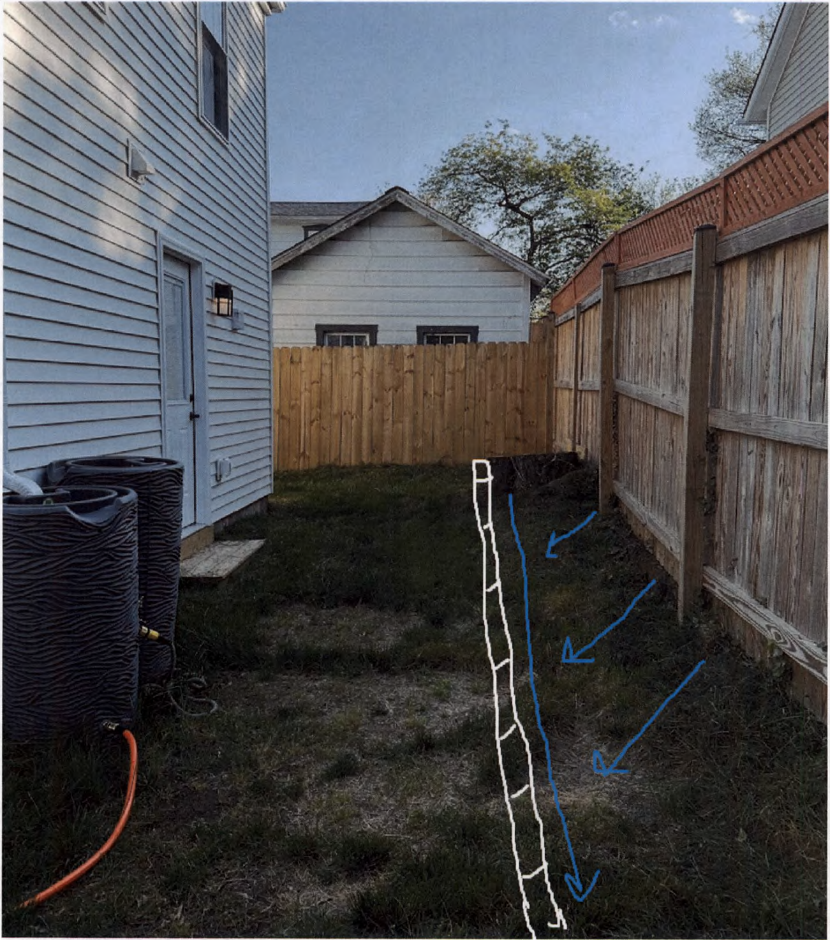
Figure 5: Stormwater that enters downslope through or under the fence will be caught by the garden and stone wall, then diverted downslope to a gravel drain away from the foundation.
