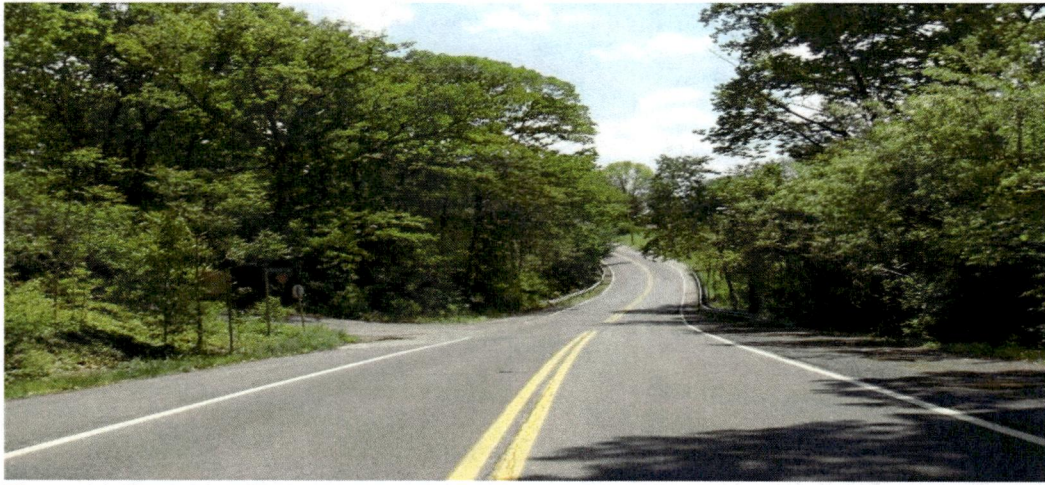
Figure 16: Transition from wide paved shoulder to narrow shoulder on Brooklyn Bridge Road.
