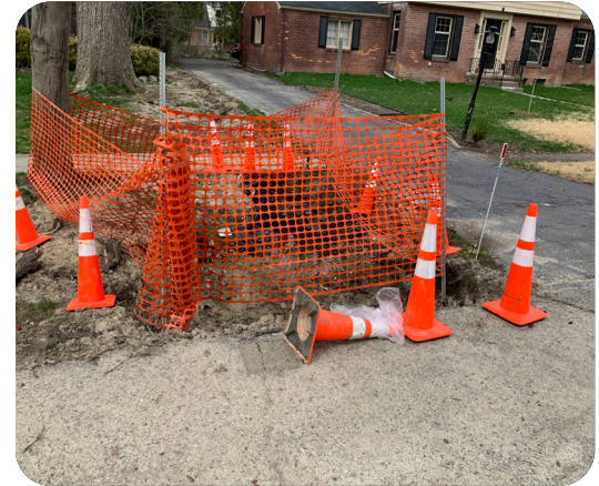
Drainage ditch repair (Giffels Webster, 2020)
