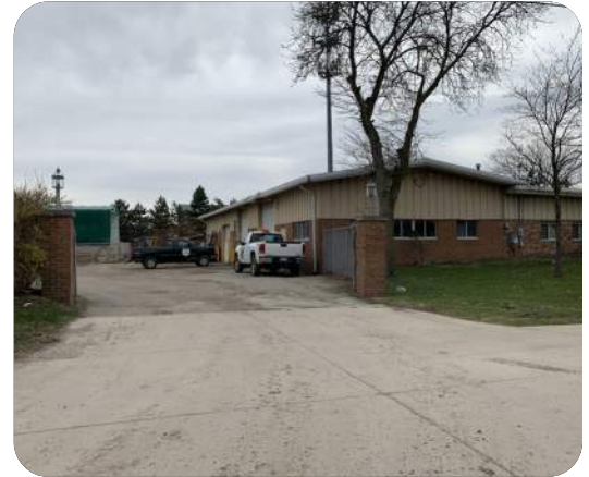
Lathrup Village DPS yard (Giffels Webster, 2020)
