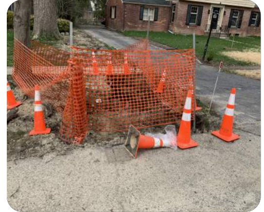
Drainage ditch repair (Giffels Webster, 2020)
