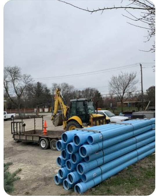
Lathrup Village DPS yard (Giffels Webster, 2020)
