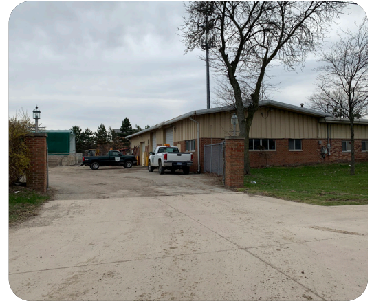
Lathrup Village DPS yard (Giffels Webster, 2020)
