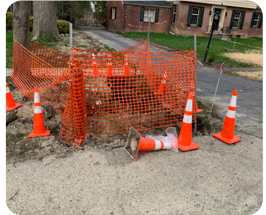
Drainage ditch repair (Giffels Webster)
